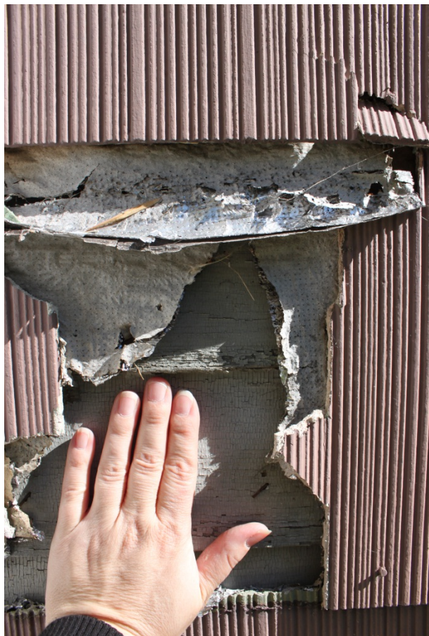
Exposed 4" clapboard beneath cement asbestos shingle (above left), west elevation with projecting bay (above right), and blocked-in windows on south elevation (below)
