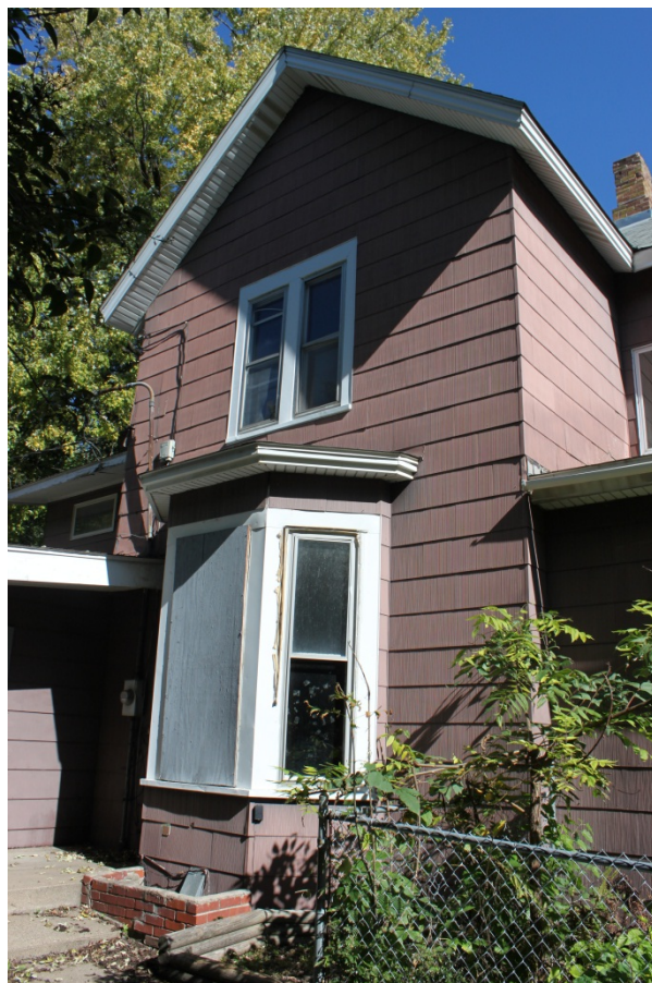
Exposed 4" clapboard beneath cement asbestos shingle (above left), west elevation with projecting bay (above right), and blocked-in windows on south elevation (below)
