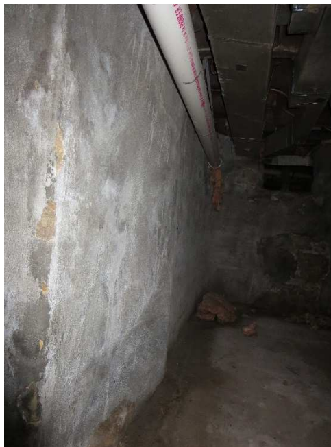
Picture 7 – Interior Foundation Walls
