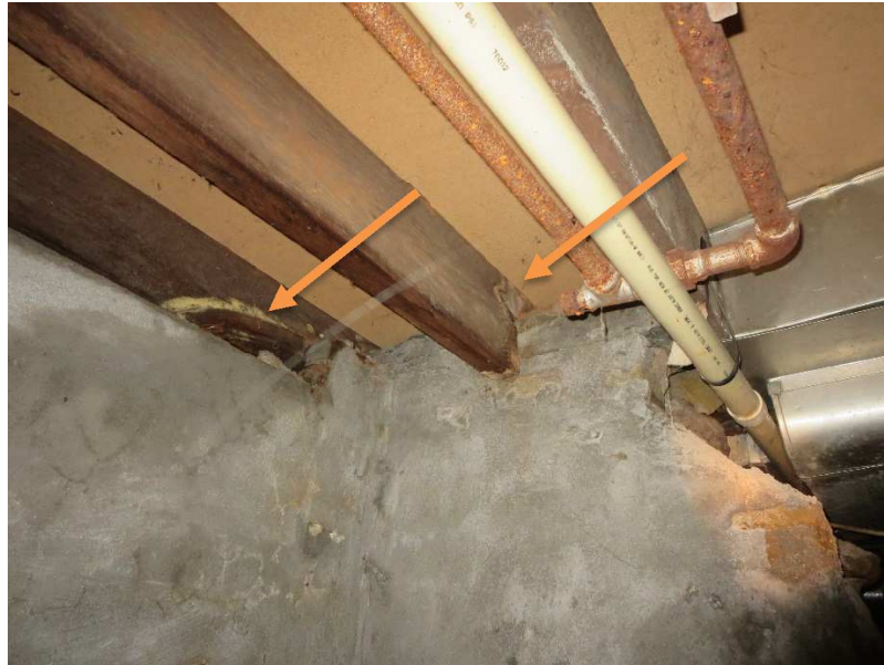
Picture 5 – Joists Bearing on Foundation Wall
