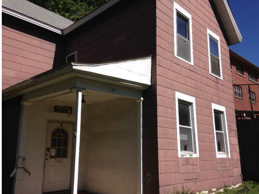
Picture 2 – Front Porch
