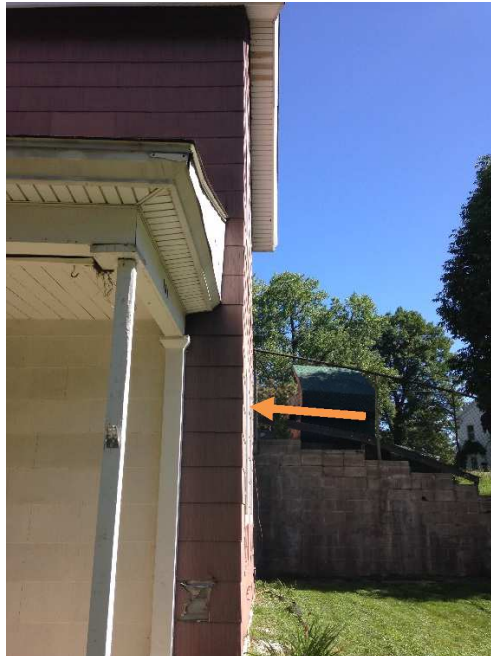
Picture 9 – House Exterior Wall
