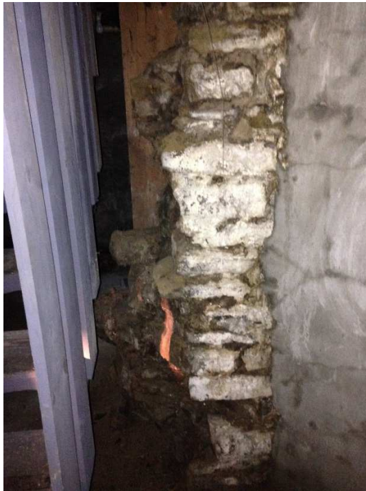
Picture 6 – Interior Foundation Walls
