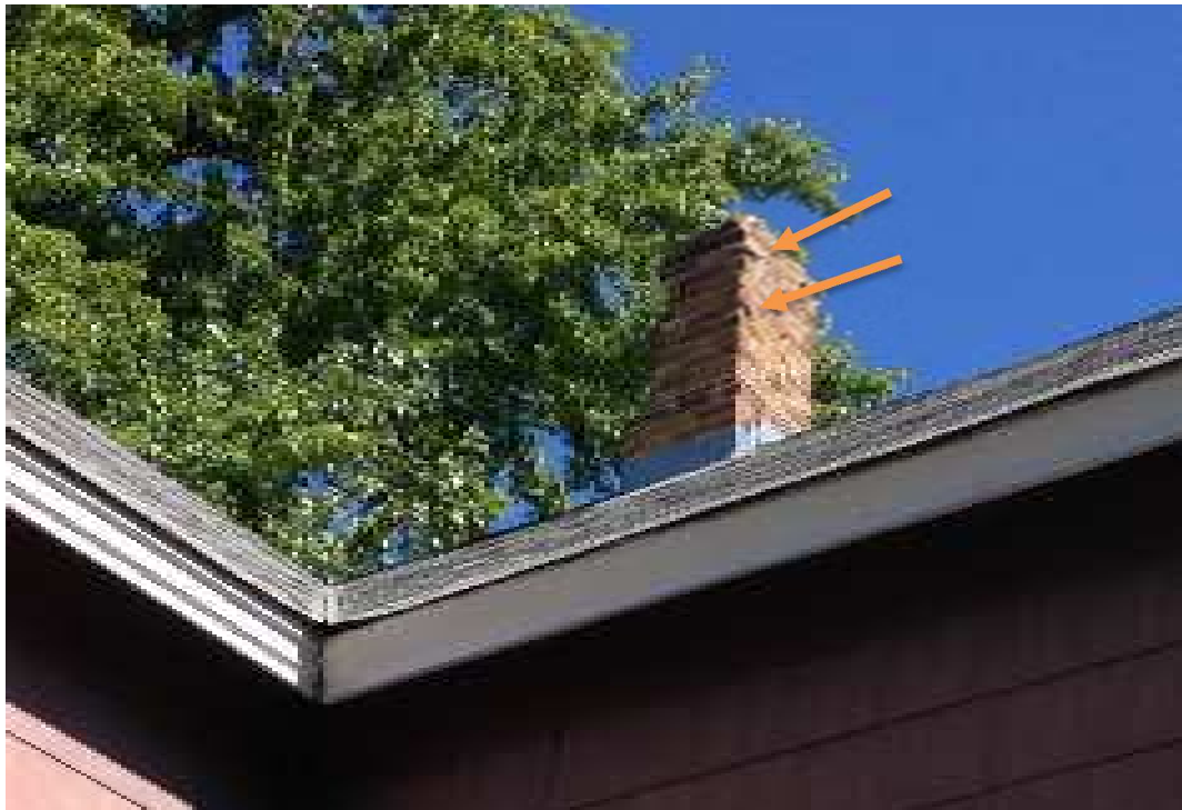
Picture 3 – Chimney in Center of House
