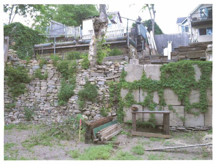
ONTHERIGHT ARE THE CONCRETE TAILINGS (BLOCKS) THAT WE HAD INSTALLED TO PREVENT SOIL EROSION IN OUR BACKYARD (AT LEAST 10 YEARS AGO).
