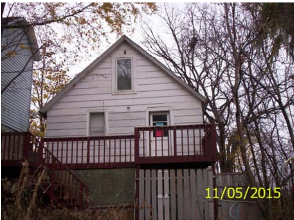
South side, posting
