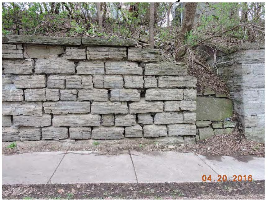
Delamination of limestone face
