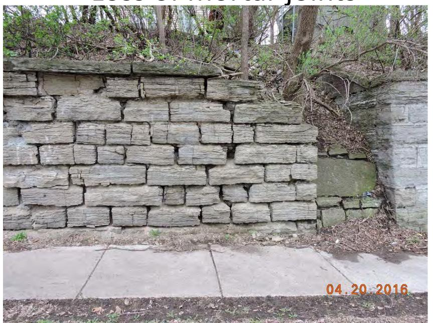
Delamination of limestone face
