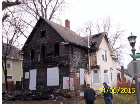
South and east sides, posting
