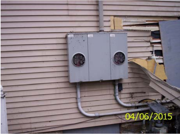
Electric meters pulled
