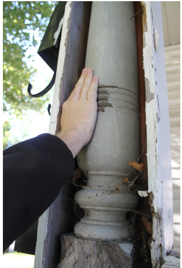
Exposed section of enclosed turned spindlework from original front porch (above), south wall of front room looking into enclosed front porch (below)
