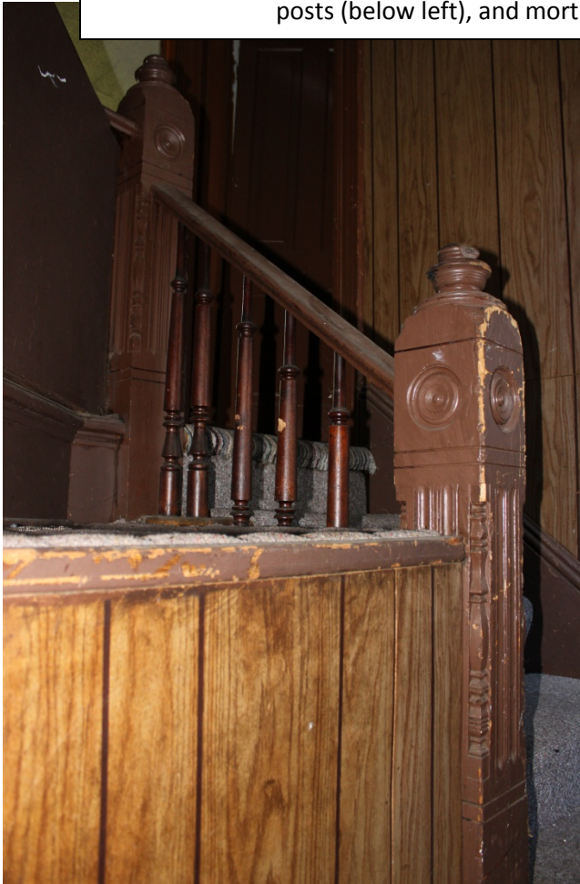
Basement conditions (above), exposed section of original Eastlake style balusters and newel posts (below left), and mortise & tenon detail of upstairs door.
