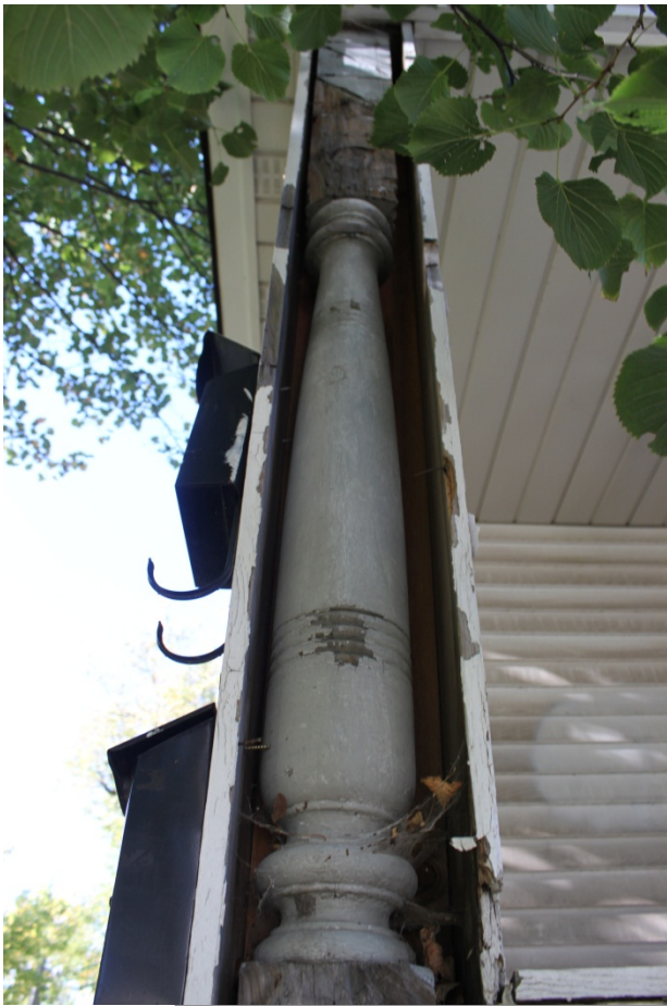
Exposed section of enclosed turned spindlework from original front porch (above), south wall of front room looking into enclosed front porch (below)
