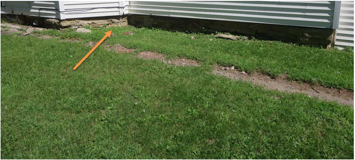
Picture 13 – Foundation Deterioration
