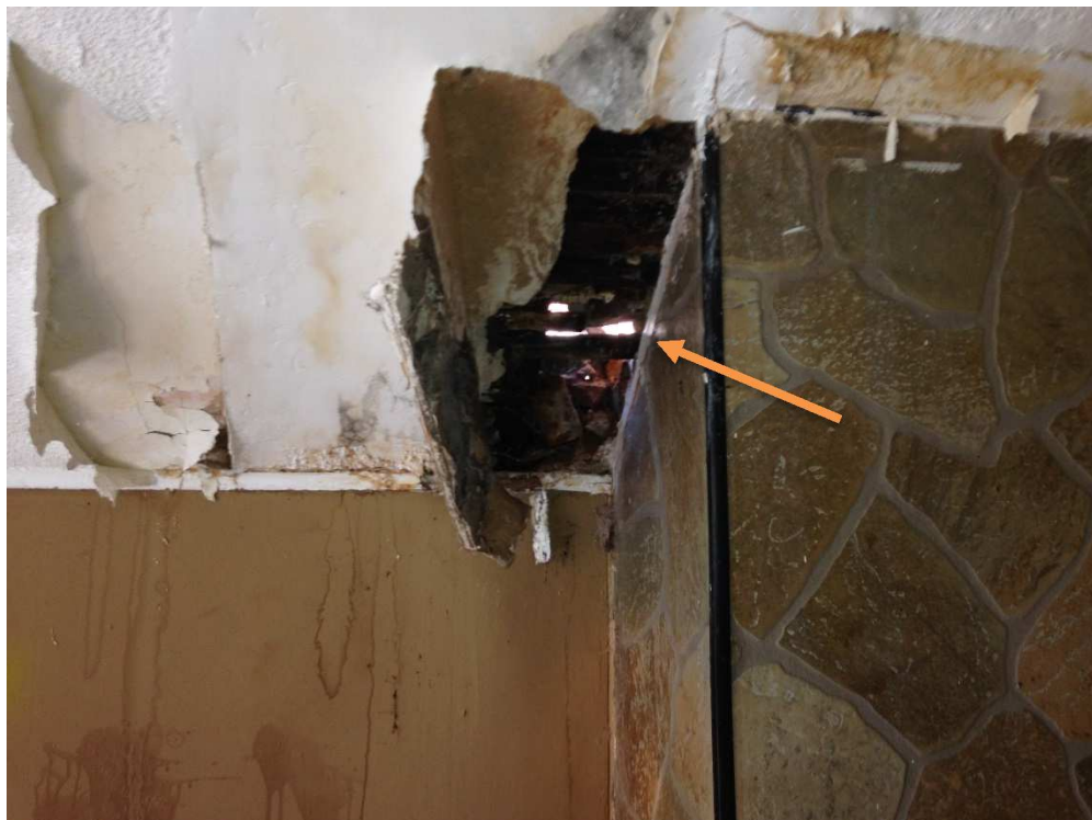
Picture 11 – Rot Through Roof
