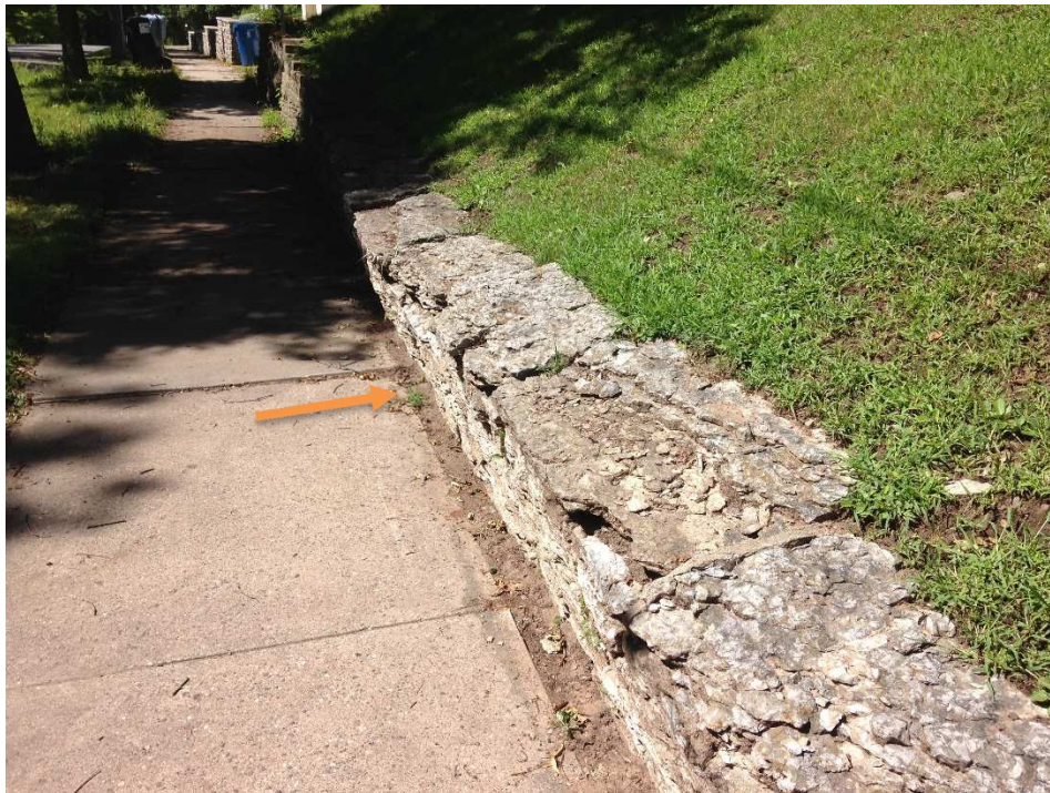
Picture 1 – Front Retaining Wall
