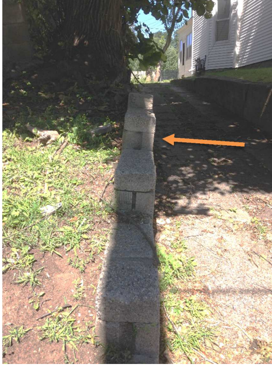
Picture 2 – East Retaining Wall
