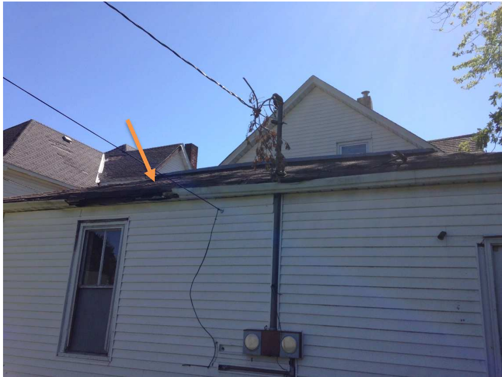
Picture 10 – Rot At Back Roof
