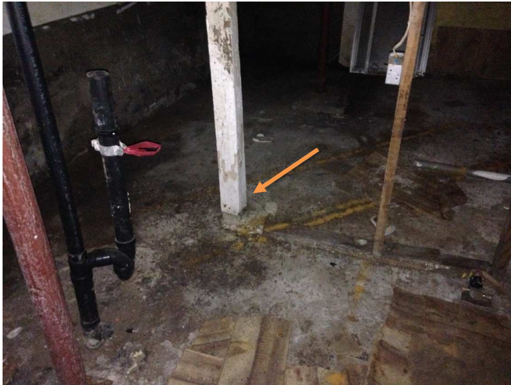
Picture 15 – Basement Column and Footing
