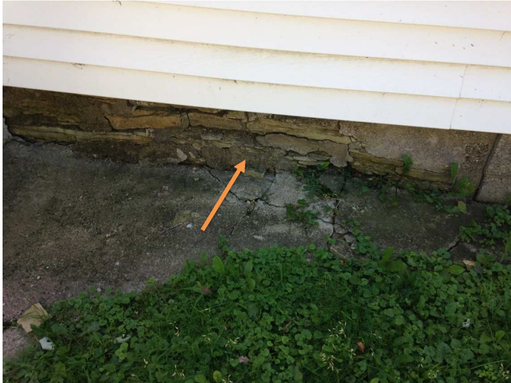
Picture 12 – Foundation Deterioration
