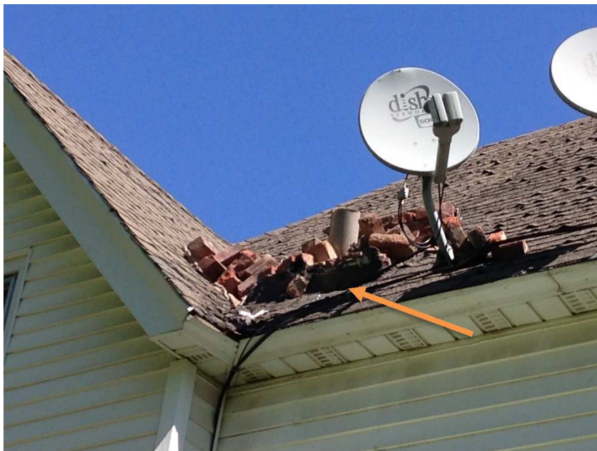
Picture 7 – Demolished Chimney
