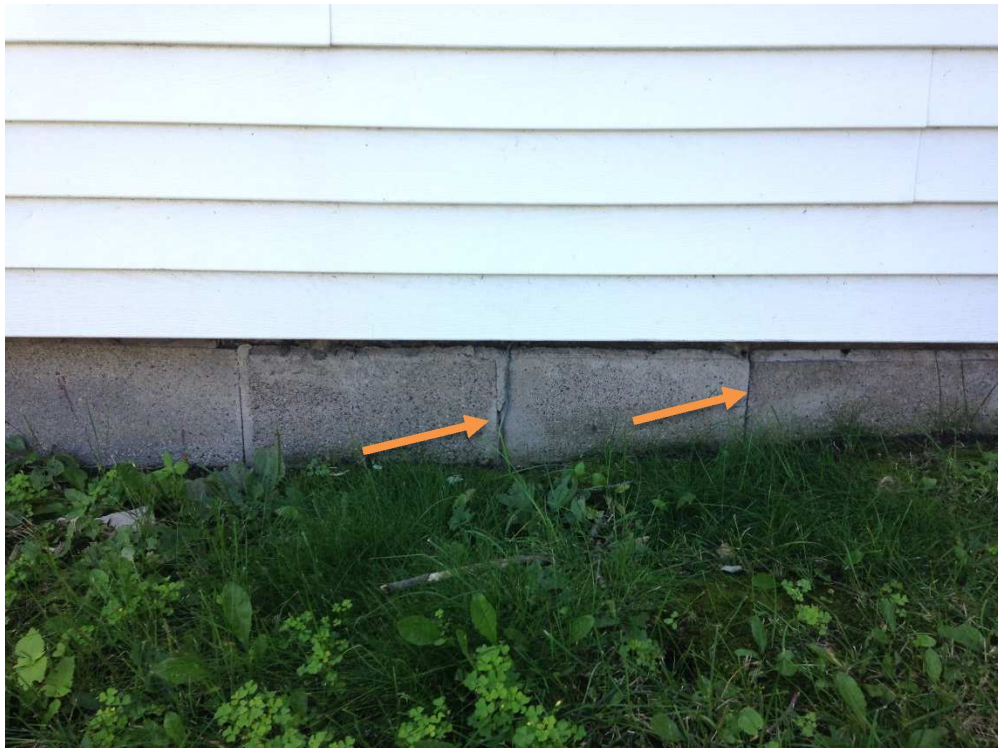
Picture 14 – No Mortar Between CMU Units
