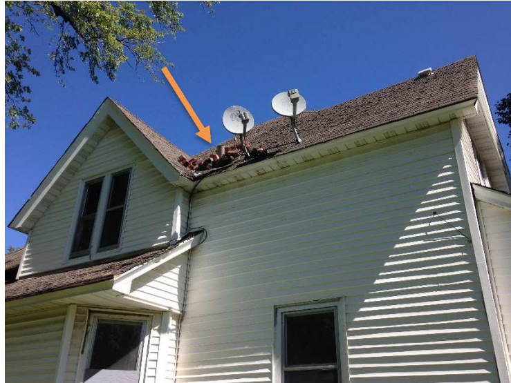
Picture 6 – Demolished Chimney
