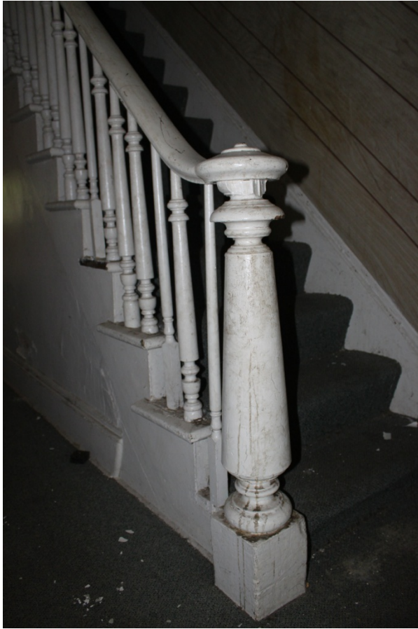
Front stairwell balusters and newel post (above), trim detail in front hall (below left), and east elevation projecting bay window in Dining Room (below right)
