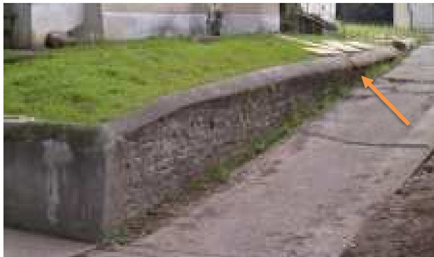
Picture 3 – South Retaining Wall
