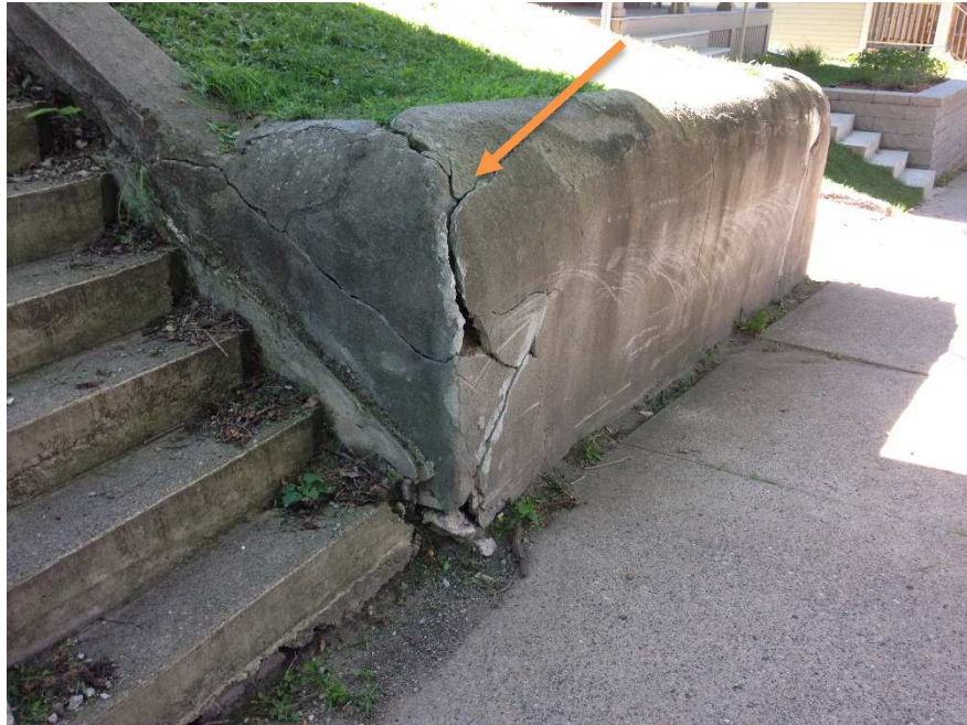
Picture 2 – Front Retaining Wall
