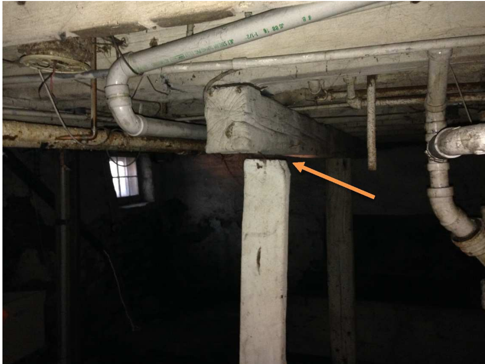
Picture 9 – Beam Above Column in Basement
