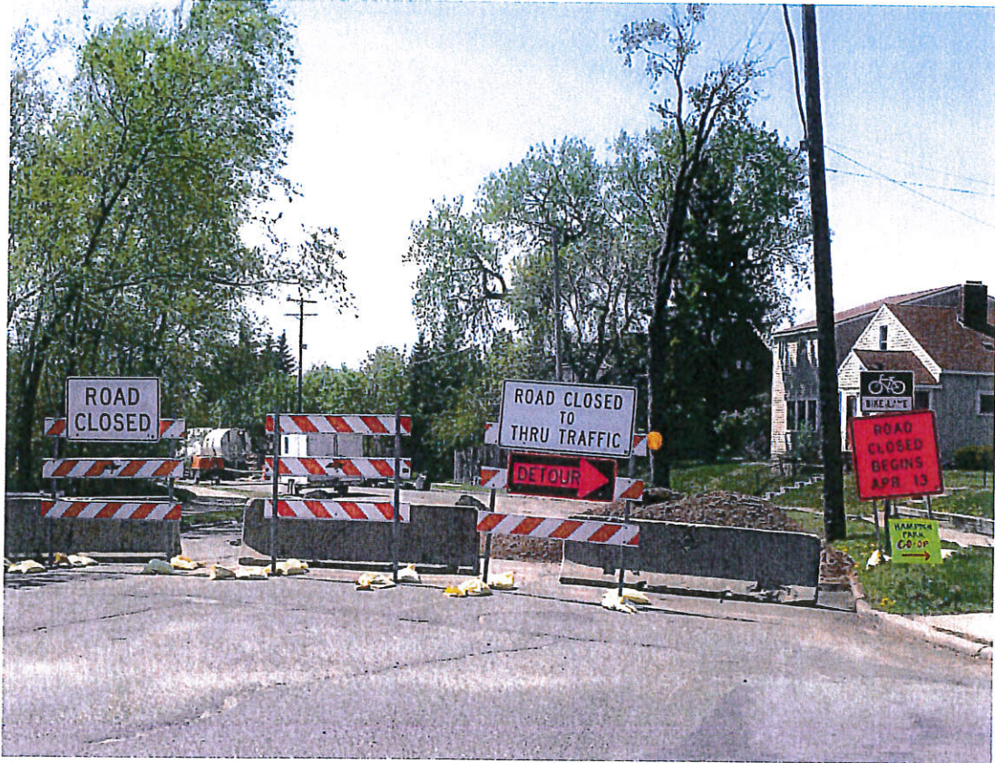
5) Road closed at Raymond Ave and Manvel Street for construction.
