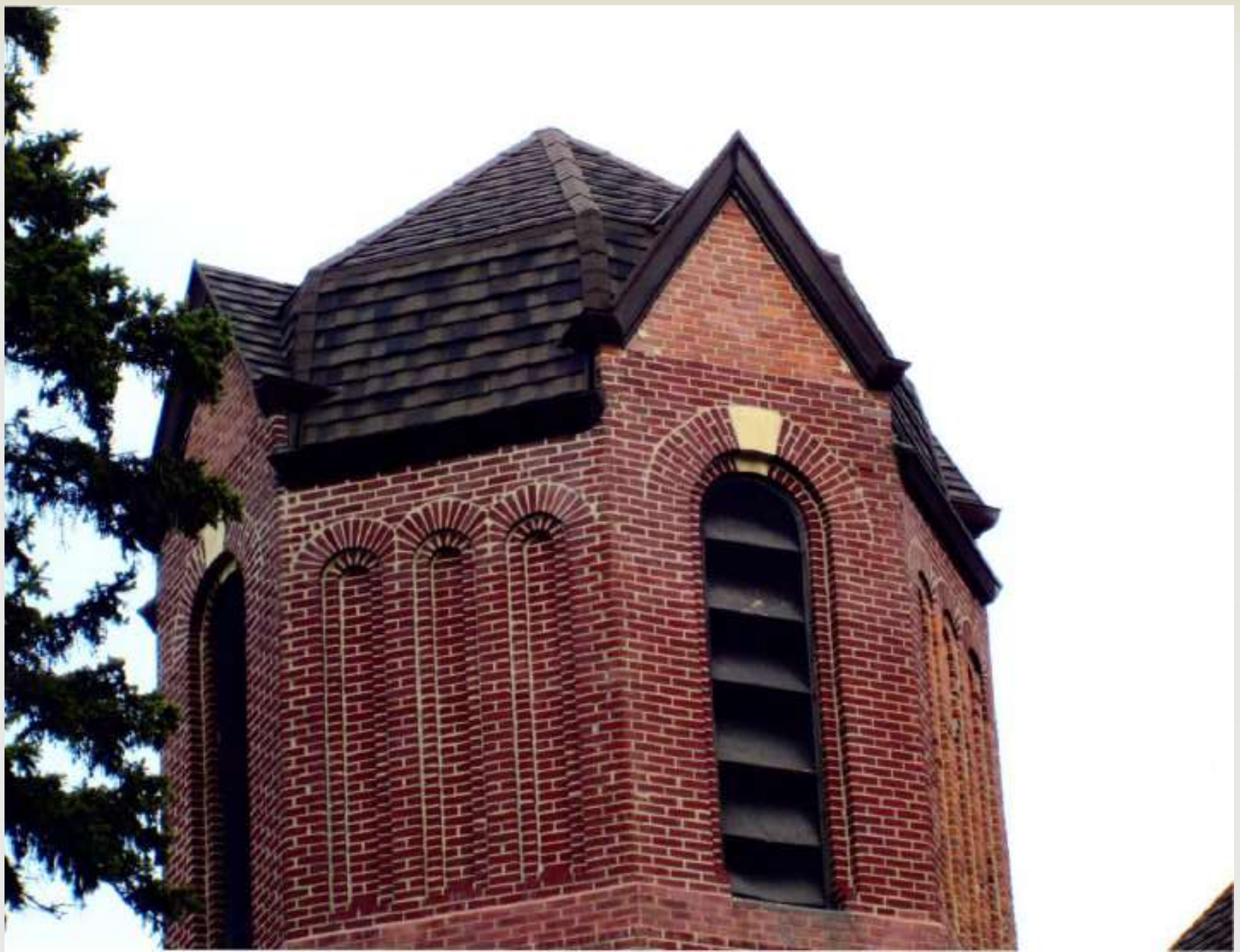
Figure 2 Detail of St. John Cantius Church
