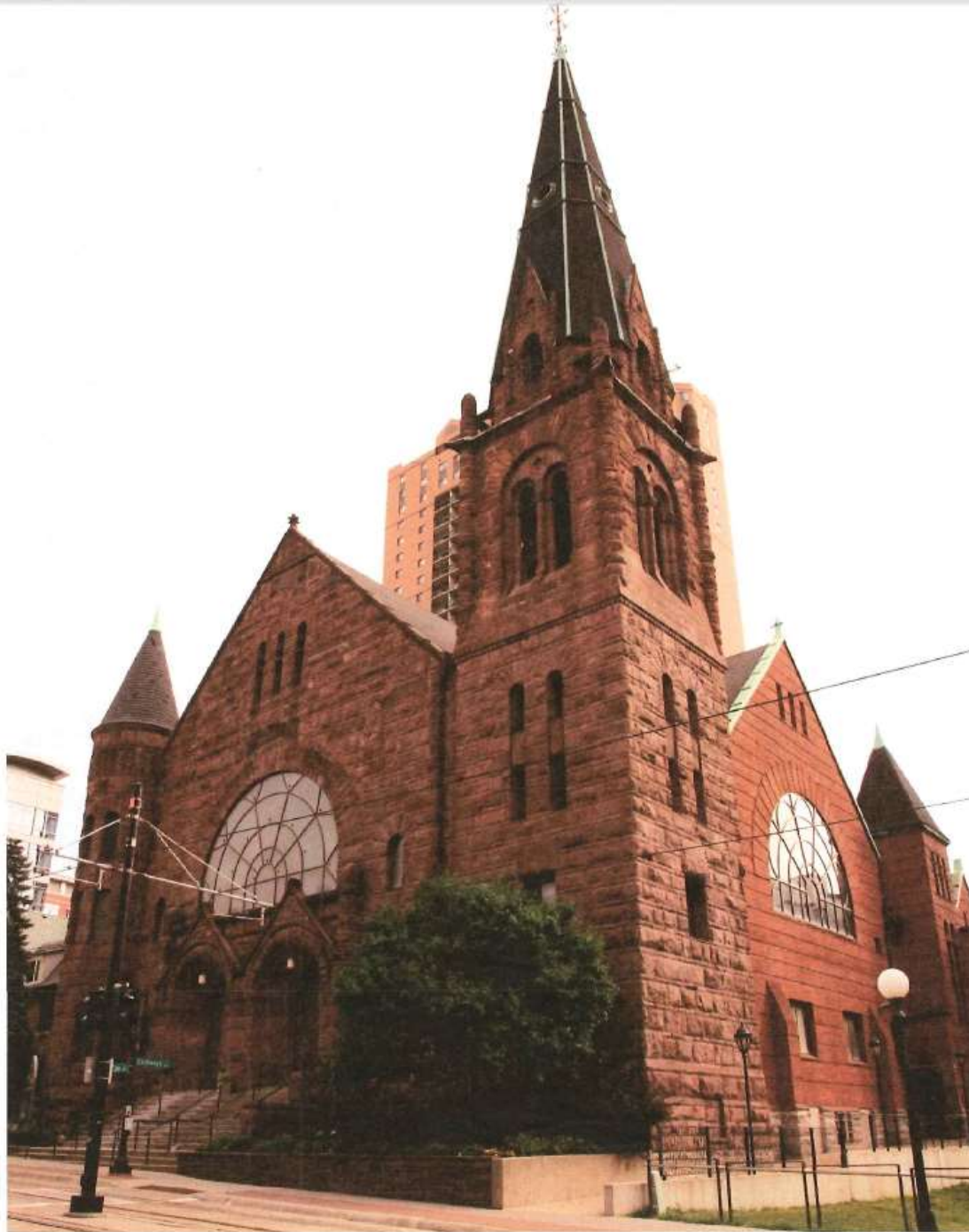
Figure 9 View taken from southwest side 7/27/15
