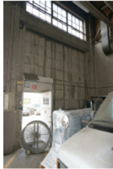
20 INTERIOR VIEW W/MAN DOOR
