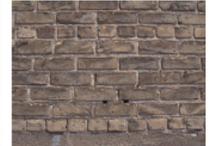
3 - SOUTH BRICK CLOSE UP
