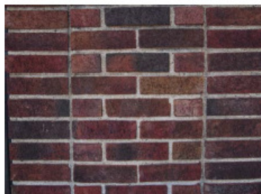
1 - North Brick Existing Building Material Palette
