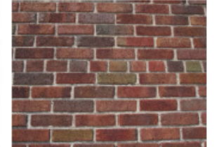
2 - EAST BRICK CLOSE UP
