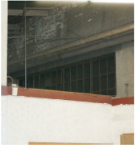
4 INTERIOR VIEW. INTERIOR COVERED UP BELOW 8'-0" A.F.F. W/ MAN DOOR
