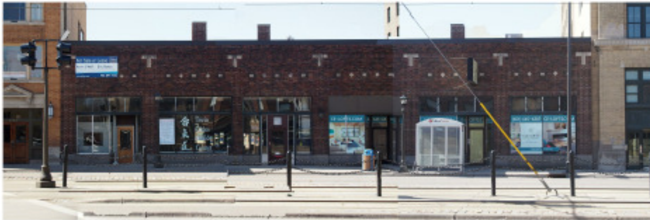
1 NORTH ELEVATION - EXISTING IMAGE 18'-10 1/2"
