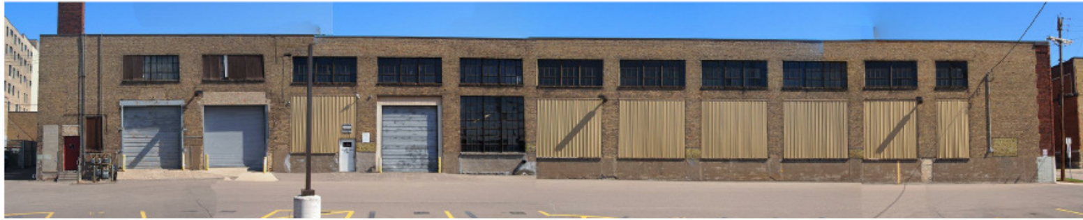
1 SOUTH ELEVATION - EXISTING IMAGE
