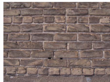
3 - South & West Brick
