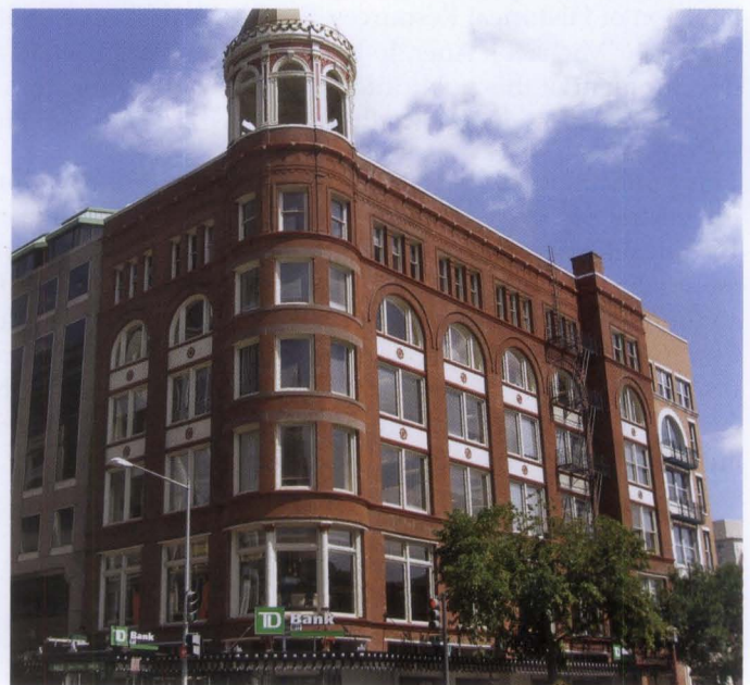
Figure 30. The small addition on the right of this late-19th century commercial structure is clearly secondary and compatible in size, materials and design with the historic building.
