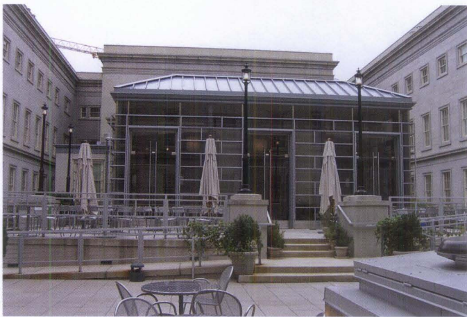
Figure 13. A glass and metal structure was constructed in the courtyard as a restaurant when this 1839 building was converted to a hotel. Although such an addition might not be appropriate in a more public location, it is compatible here in the courtyard of this historic building.
