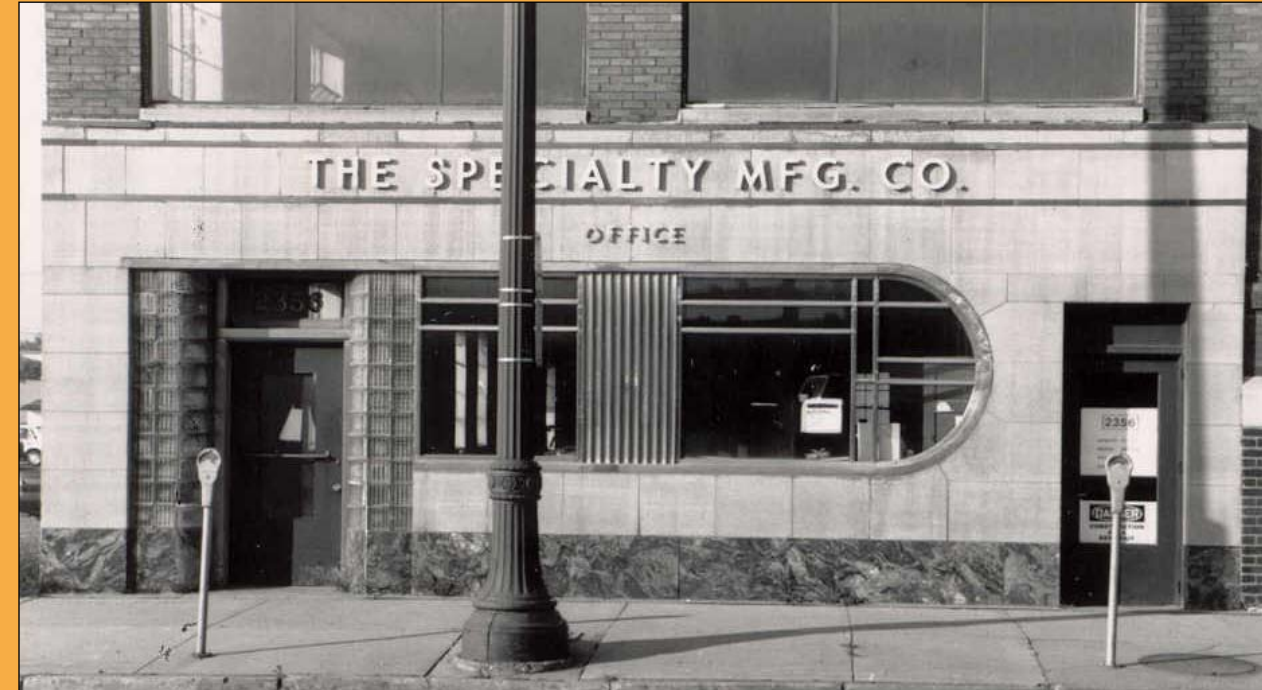
FIGURE 1.3 - Detail of the Specialty Manufacturing Company, built 1906.
