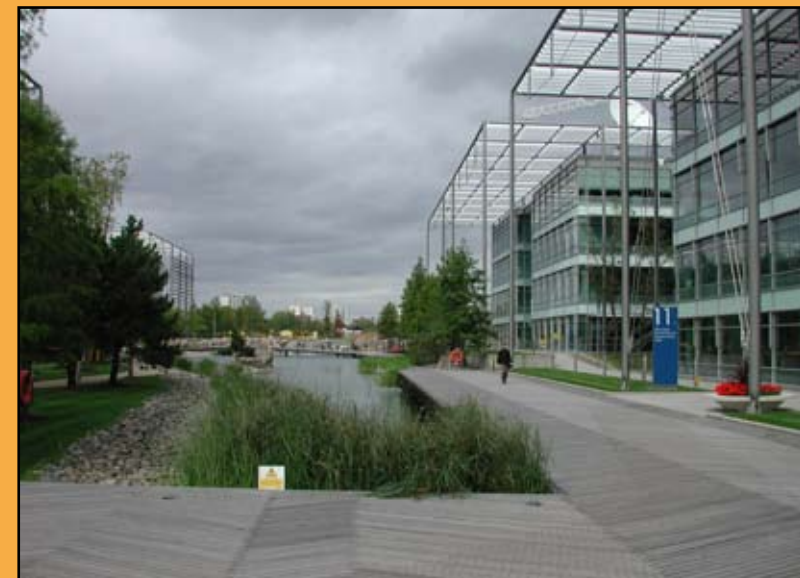
FIGURE 4.5 - A large open space with integrated stormwater management helps to provide structure and create a prestige address for this employment district in London, UK.
