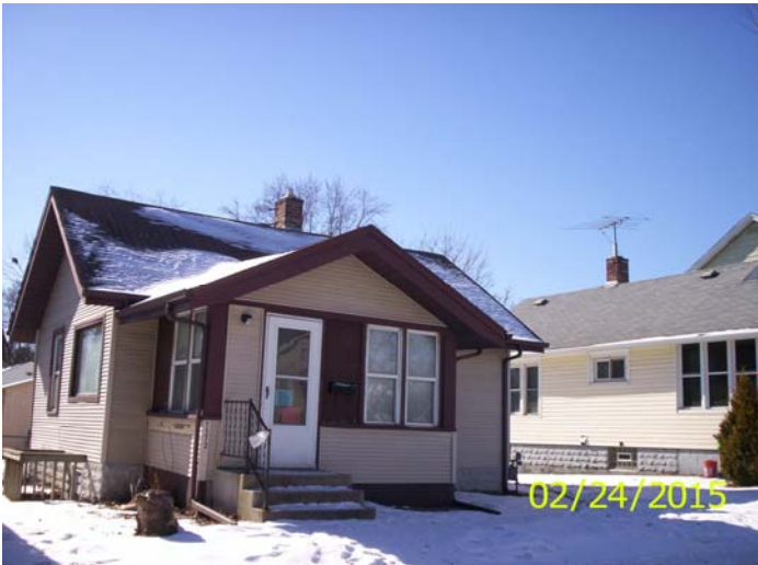
North and east sides, posting
