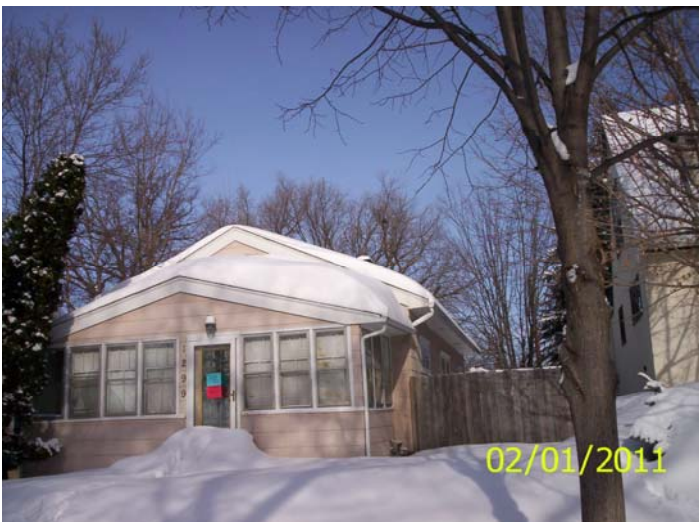
South and east sides, posting
