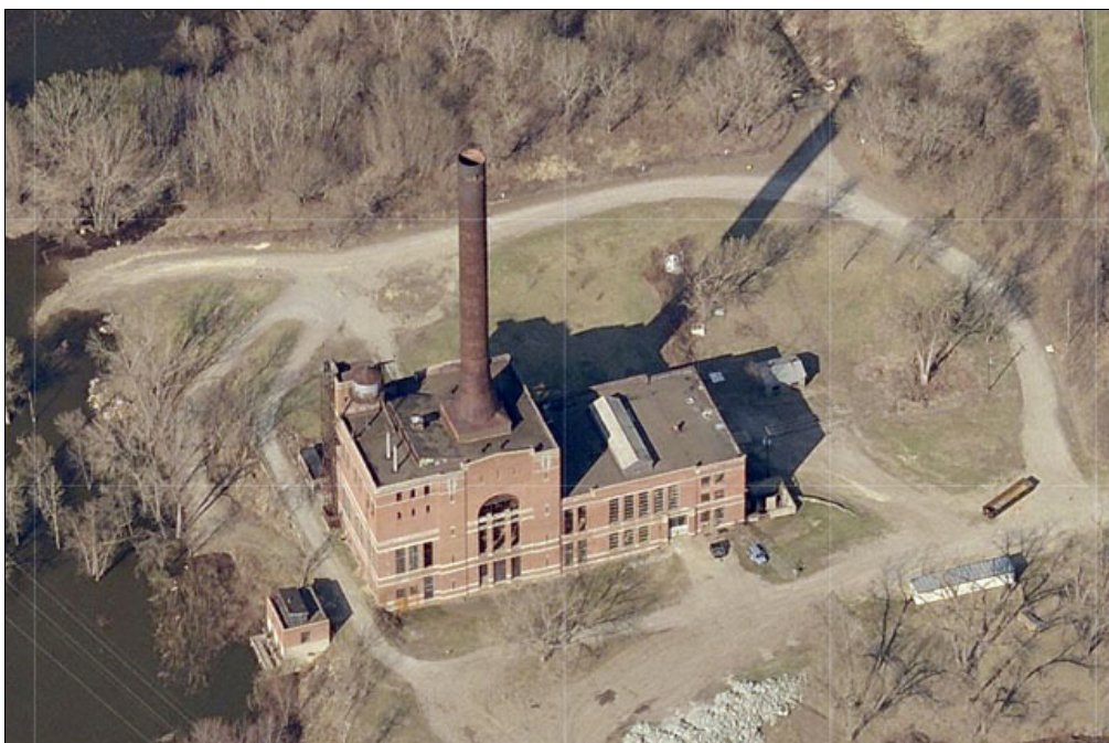
Figure 8. Island Station, looking northwest, 2012. (Bing)
