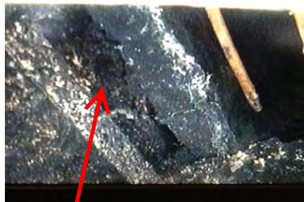
Gaps around the bricks and the bottom flue tile in main level smoke chamber
