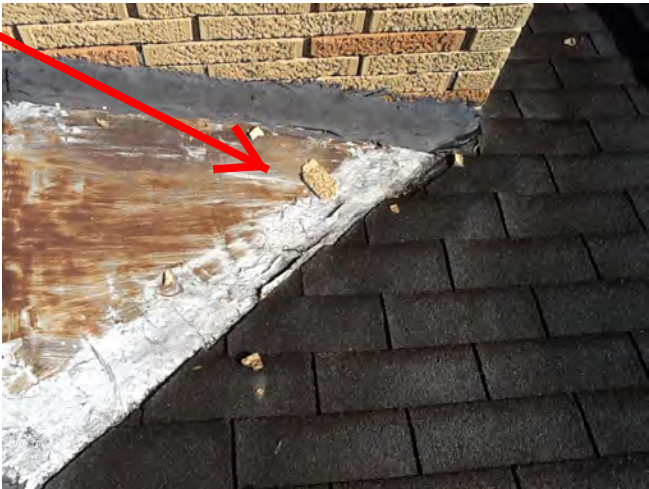
Spalling brick and deteriorating mortar joints
