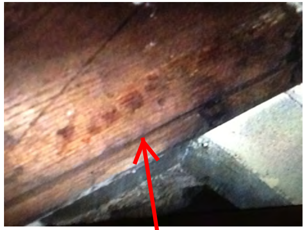
Wood in ash dump of main level fireplace
