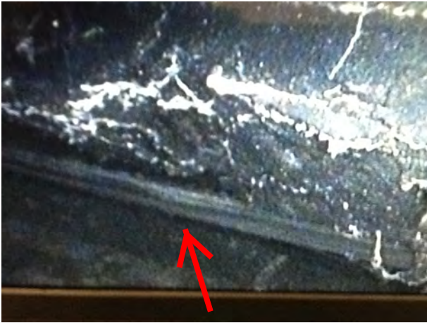
Wood in lintel area main level fireplace
