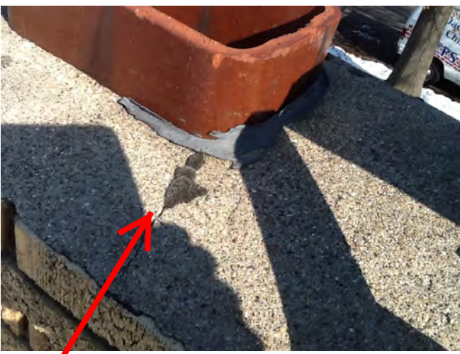
Cracks in wash at the top of the chimney
