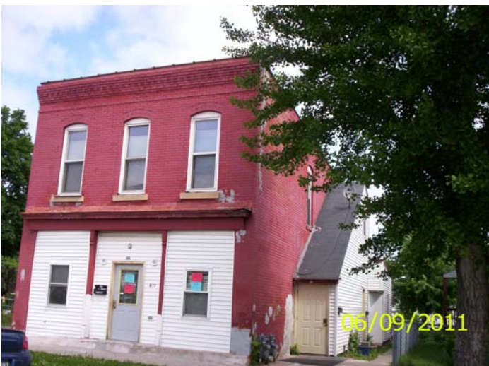
South and east sides, postings
