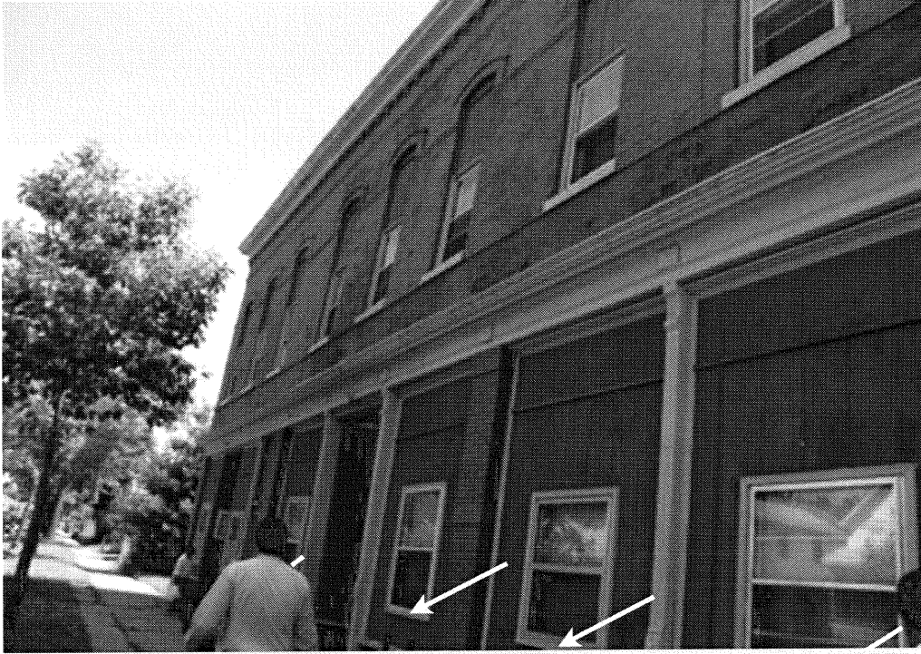
Four (4) of the nine (9) window sills that will be repaired or replaced are shown here.
