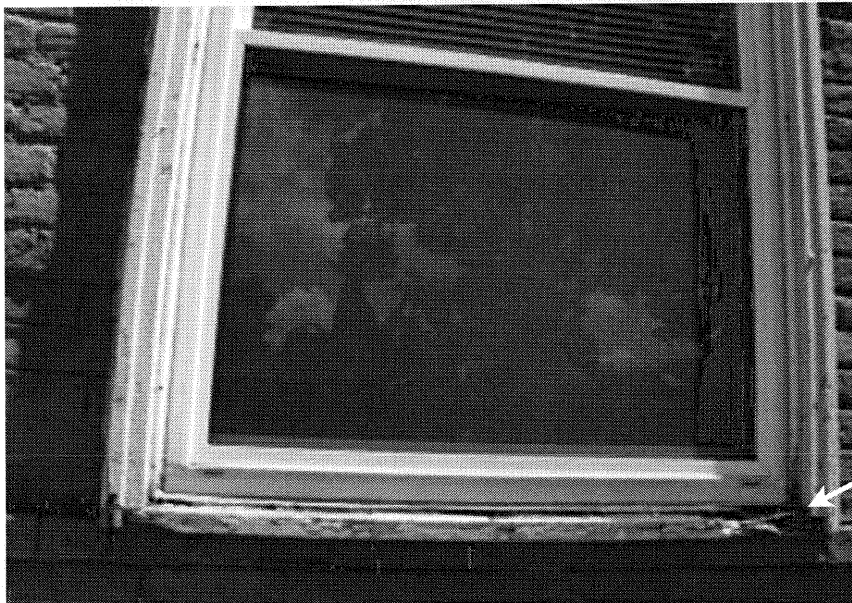
Nine (9) of the window sills must be patched or repaired. The one here needs to be replaced.
