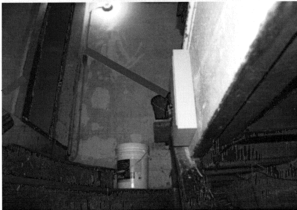
One handrail to be installed at the top of stairs, 36 inches above stairway
