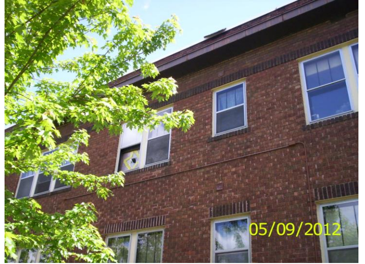
Window where it appears work is being done
