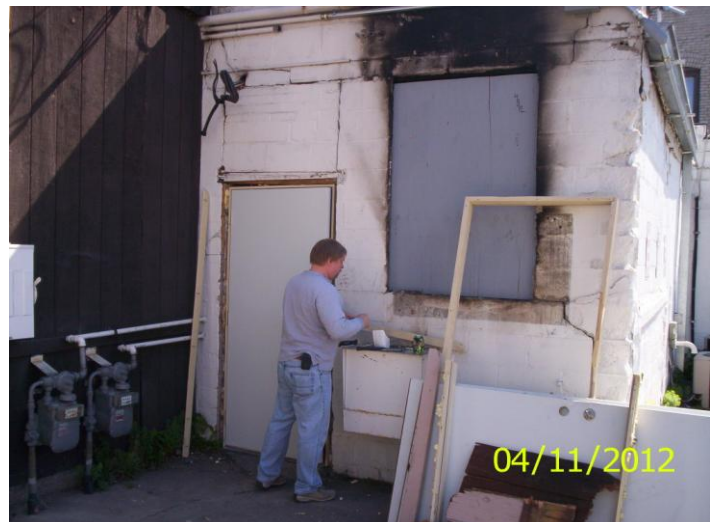
South side door and window
