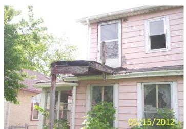
Deteriorated and missing 2<sup>nd</sup> floor porch/steps/rails
