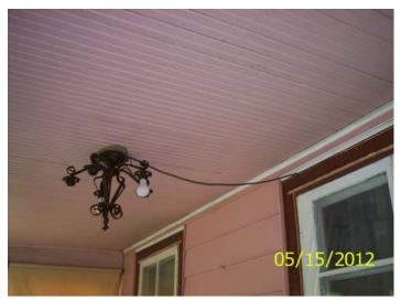
**Extension cord wiring to light fixture**
