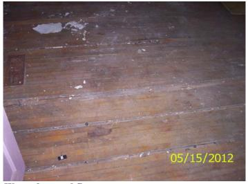
Water damaged floor
