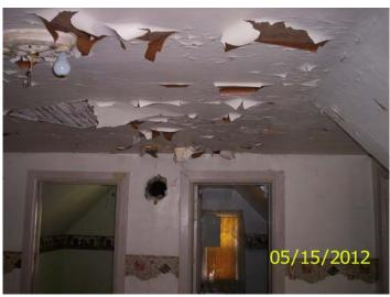
Water damaged ceiling, open chimney
