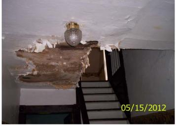
Water damaged ceiling
