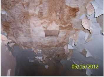
Water damaged ceiling
