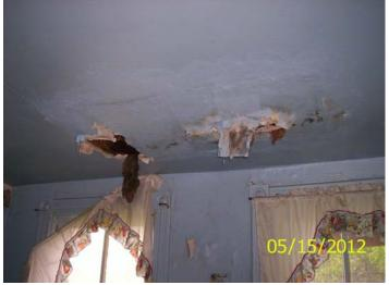
Water damaged and partially collapsed ceiling
