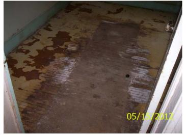
Water damaged floor
