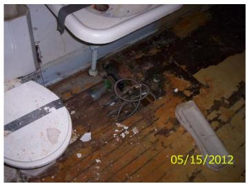
Water damaged floor
