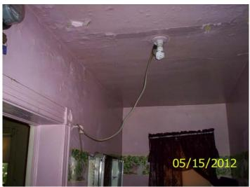
Extension cord wiring to light fixture
