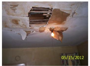
Water damaged and partially collapsed ceiling
