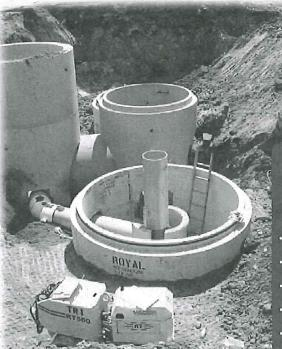
ecoStorm® design allows for tight angles between the inlet and outlet pipe. This is especially beneficial for minimizing the footprint in offline systems.
