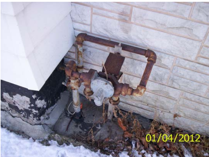
Gas meter removed
