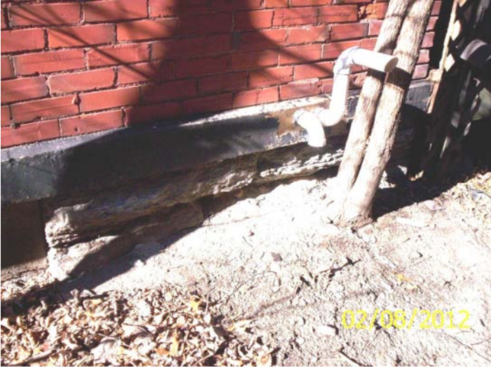
Deteriorated foundation
