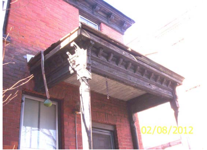
Roof over the rear deck
