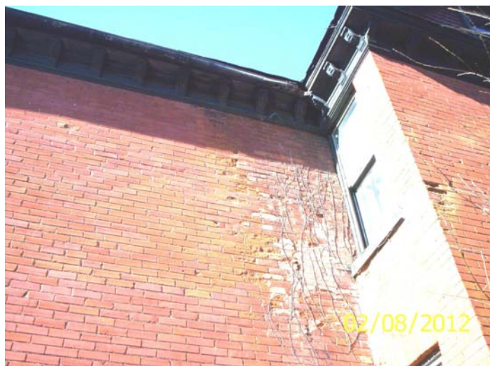
Deteriorated masonry
