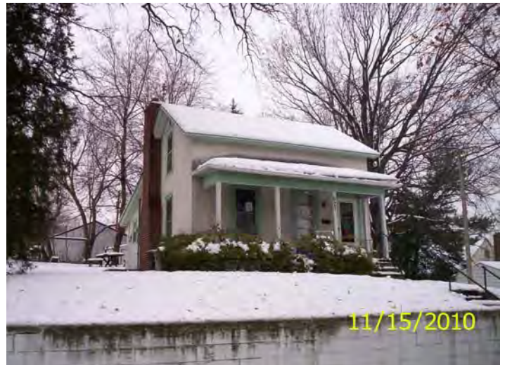
South and east sides, posting
