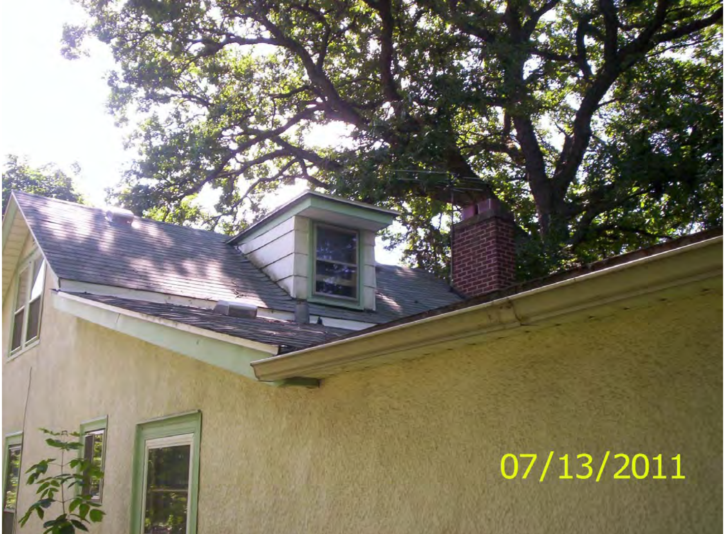
North and west face of the west side dormer, missing flashing, water damage siding
