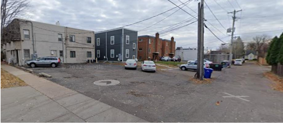
View of the property at 635 Cleveland and properties to the south from the alley
