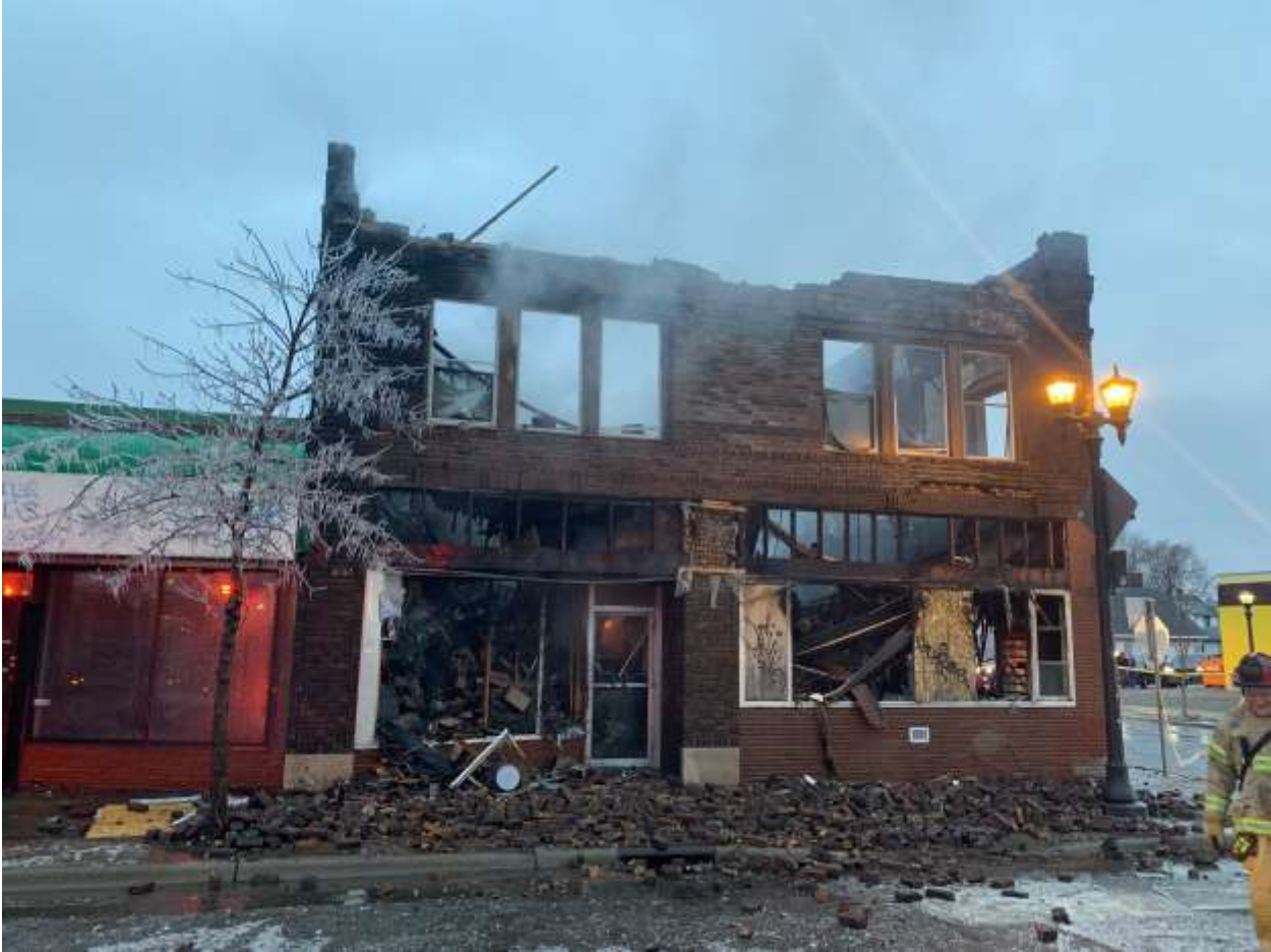
916-918 University Ave W.Fire Photos 1-10-24
