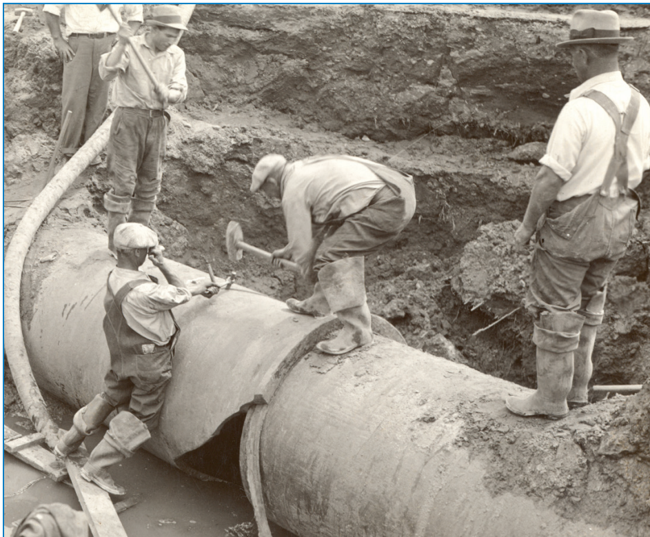
Workers make repairs on a 36-inch water-main in this undated photo. These images are part of research being done to make a
