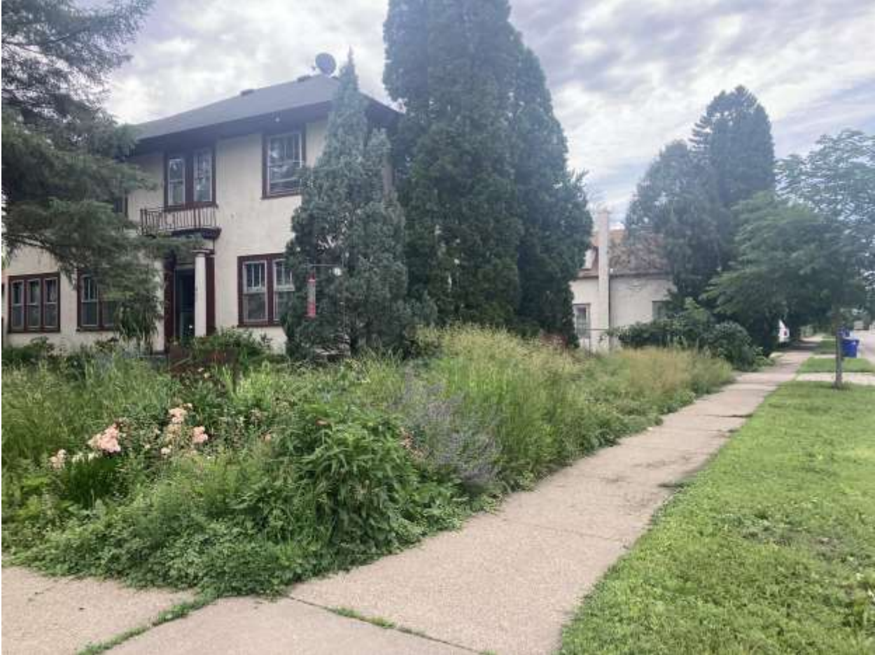
957 Flandrau St.Owner Photos.6-19-24
