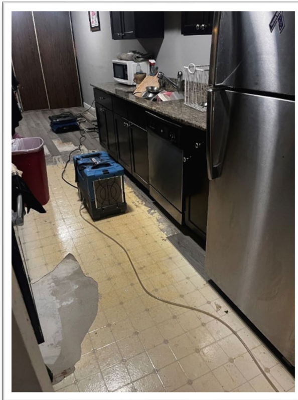
Removing presumed ACM vinyl flooring.
