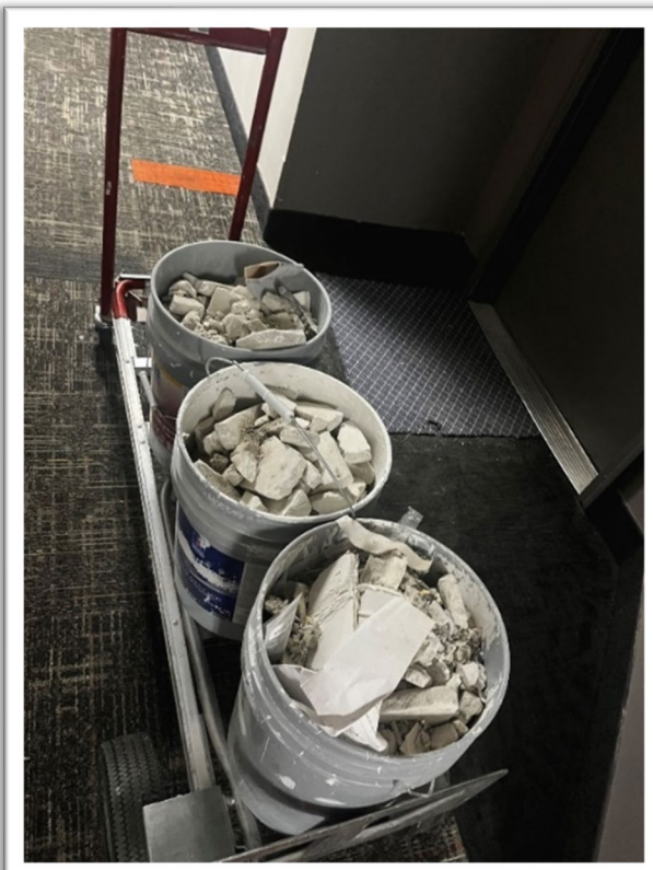
Carting uncovered suspect ACM drywall in hallways.
