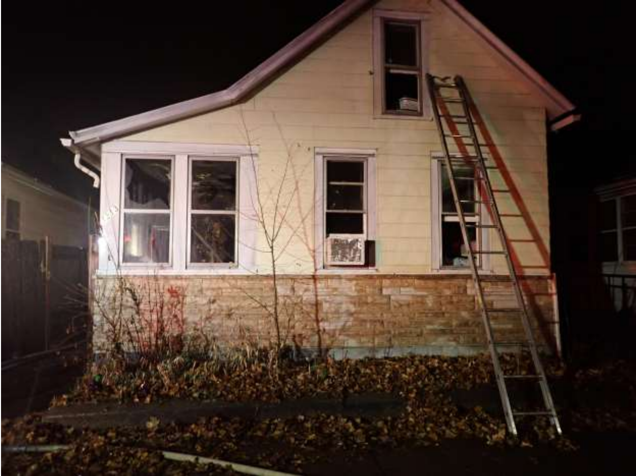
1213 Woodbridge St.Fire Photos 12-1-21
