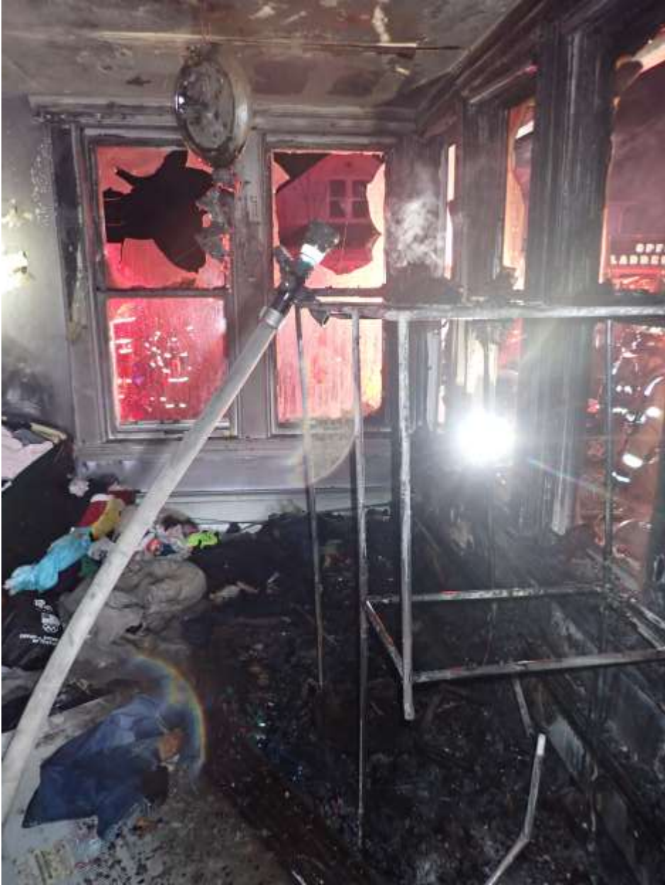
1213 Woodbridge St.Fire Photos 12-1-21
