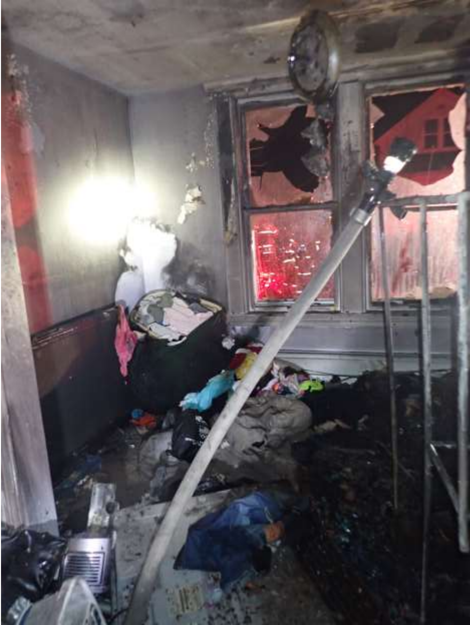
1213 Woodbridge St.Fire Photos 12-1-21
