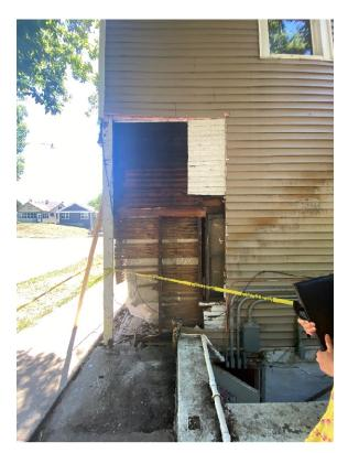
Sister new 2x4's alongside each existing member. And place on treated plate with anchor bolts per the building code. Attach at 12"
