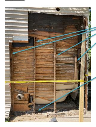
Sister new 2x4's alongside each existing member. And place on treated plate with anchor bolts per the building code. Attach at 12"
