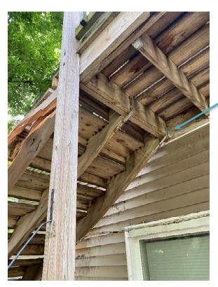
Landing pulled away from the second floor and should be re-placed
