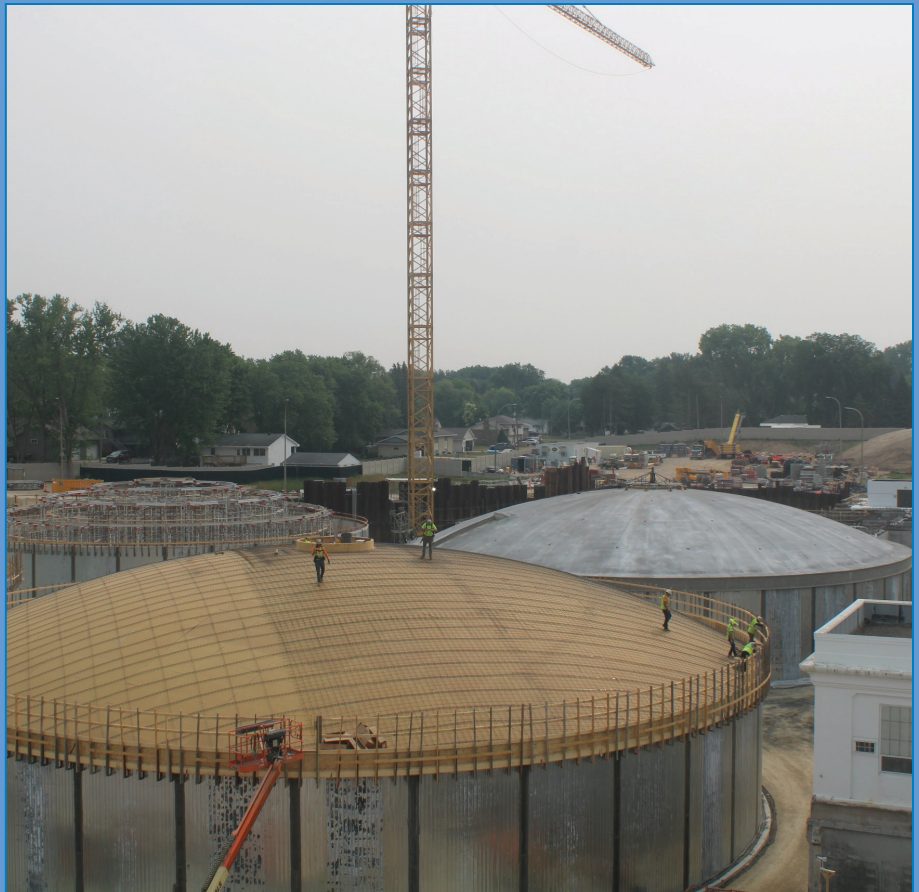
The first cover of the clarifier domes has been laid in concrete on Thursday, June 8, with the dome in the near front slated for the next concrete laying.
