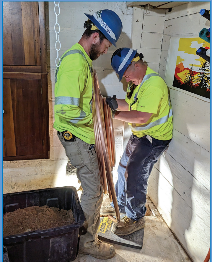
Left, Nick McBride, water system worker II, and Samuel Bartz, water utility worker I, feed copper pipe through the basement of a day care on Jessie Street on May 25.
