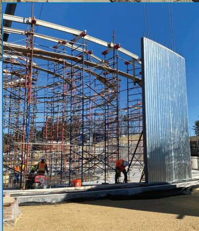
The first panels of the clarifiers going up the first week in May.
