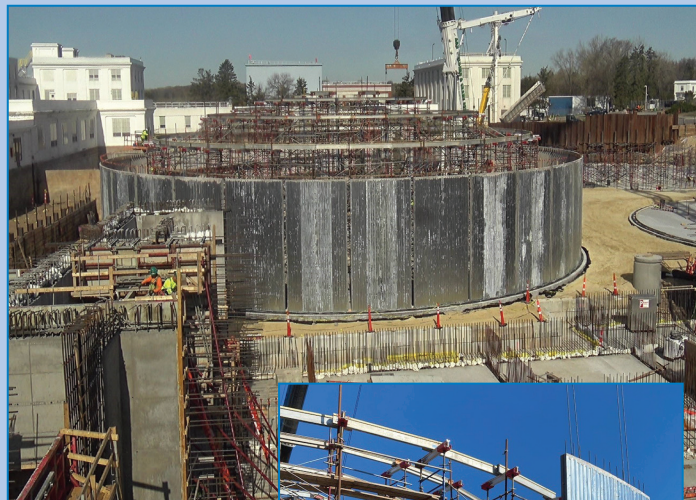
The first panels of the clarifiers going up the first week in May.
