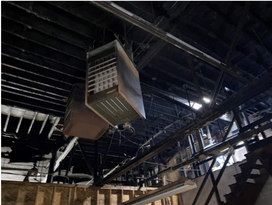
PHOTO #1: View of T1 truss near file location.
