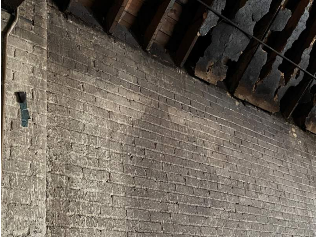
PHOTO #3: View of North Wall at T1 support column.
