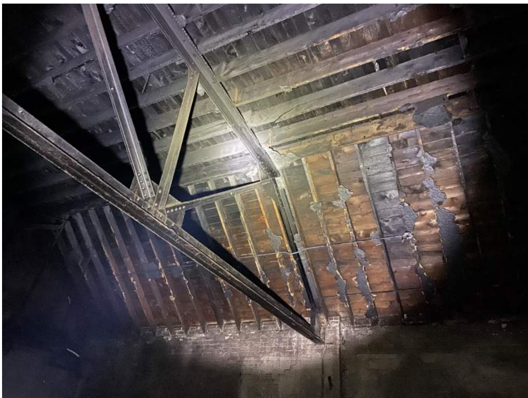
PHOTO #2: View of north end of T1 truss.
