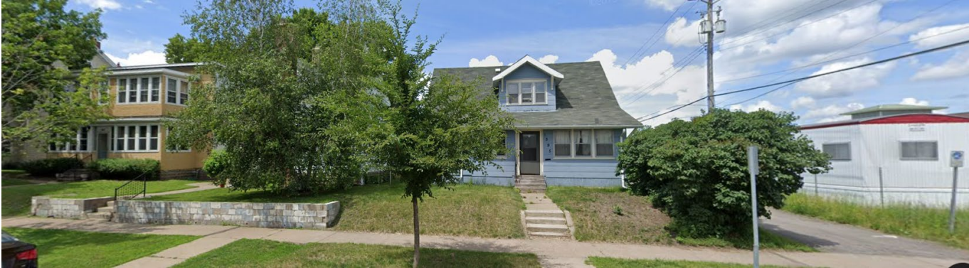
One and two-family homes north side of Carroll Avenue in RT1 district
