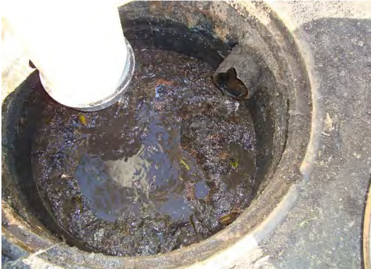
Sanitary Discharge, Private Storm Drain
