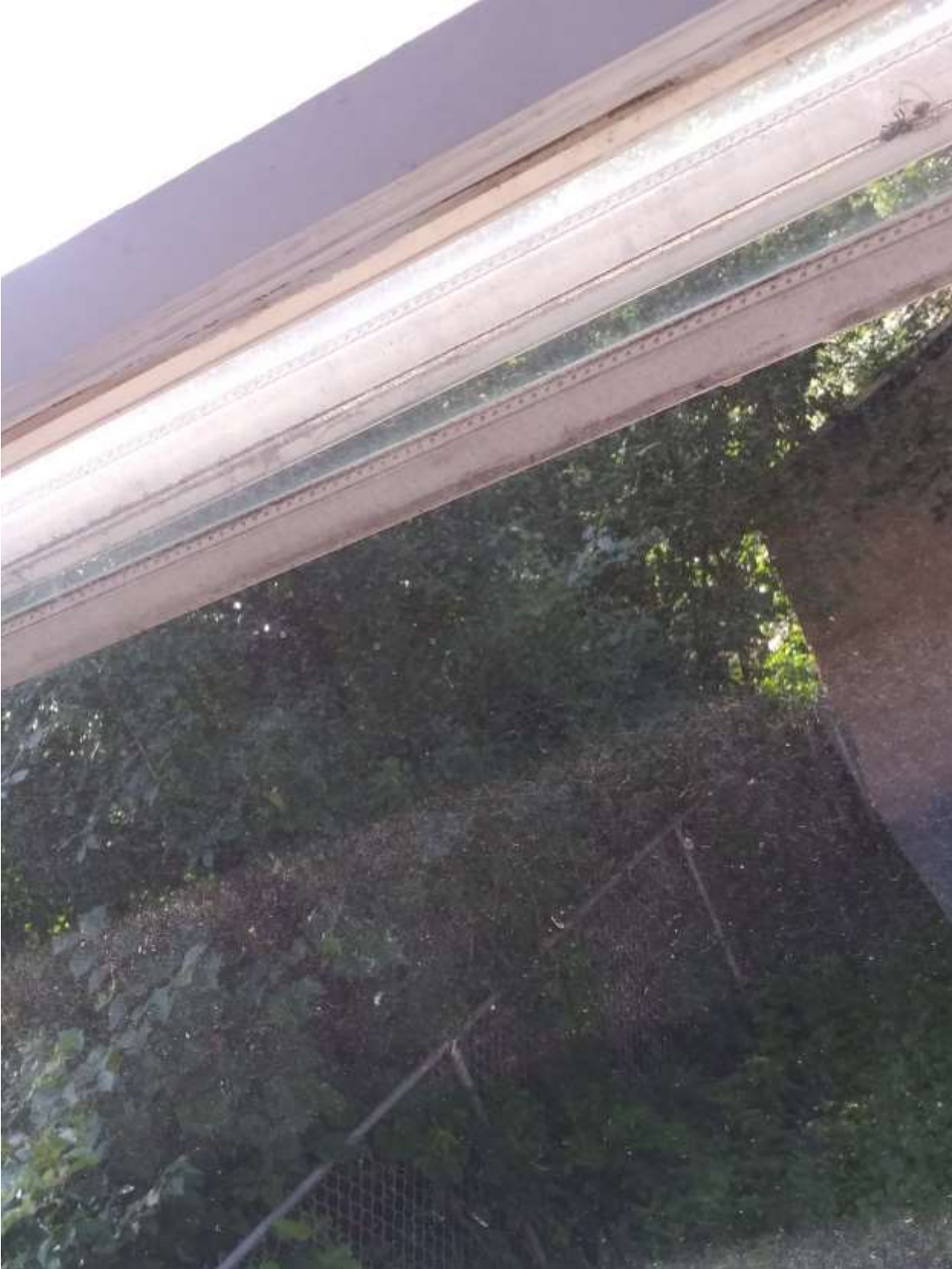
1842 Stillwater Ave. Photos sent by Lakisha Carpenter
