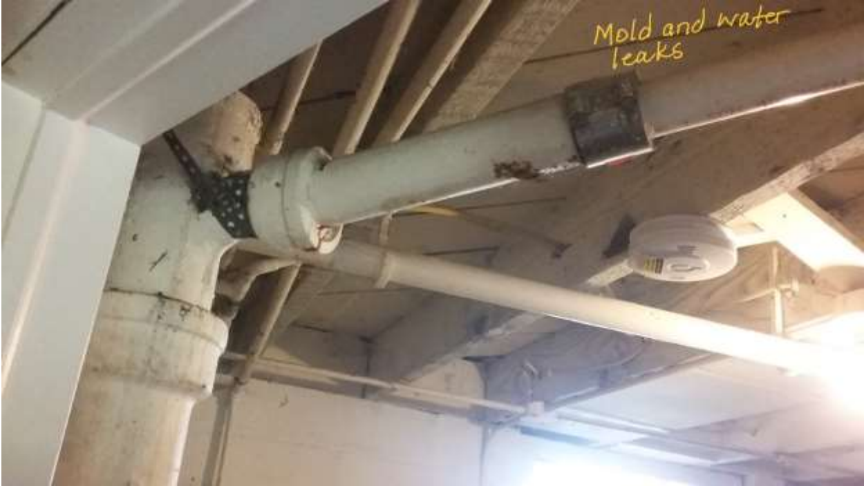
1842 Stillwater Ave. Photos sent by Lakisha Carpenter
