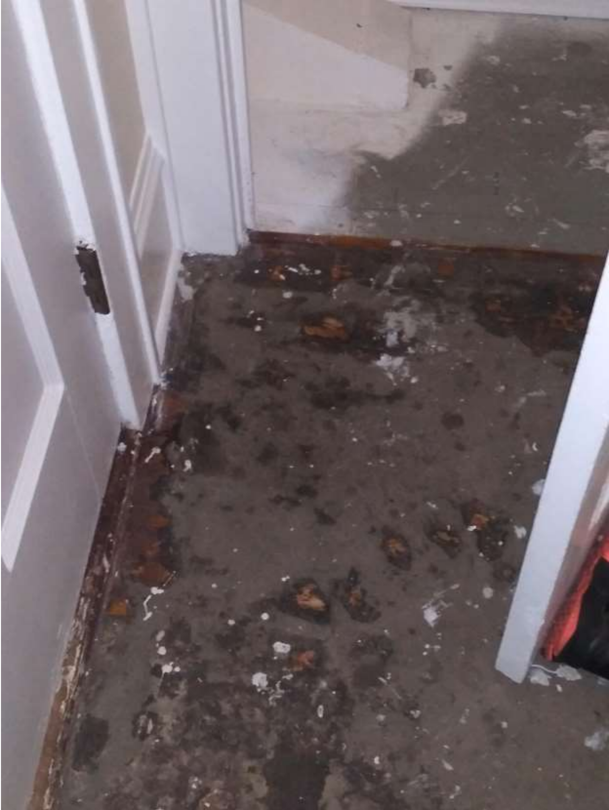
1842 Stillwater Ave. Photos sent by Lakisha Carpenter
