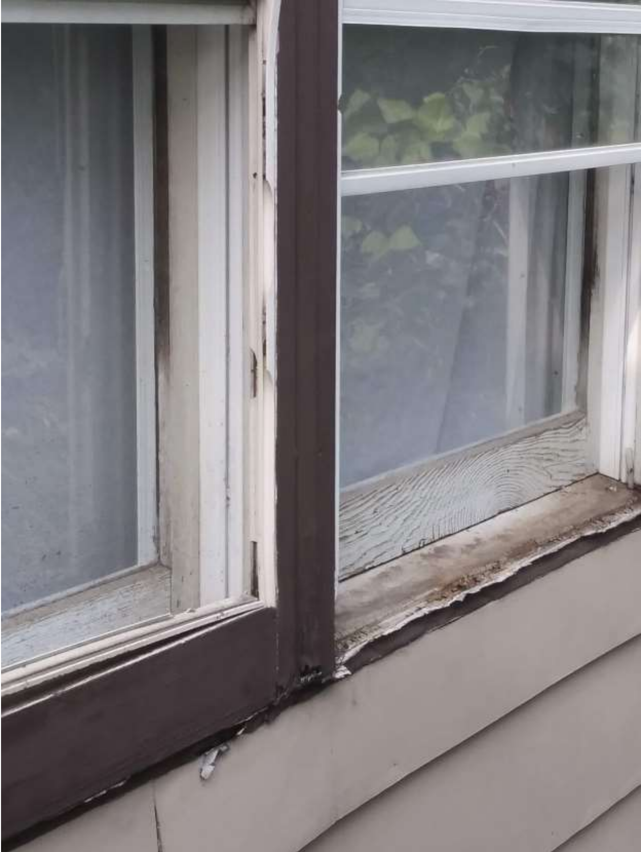
1842 Stillwater Ave. Photos sent by Lakisha Carpenter
