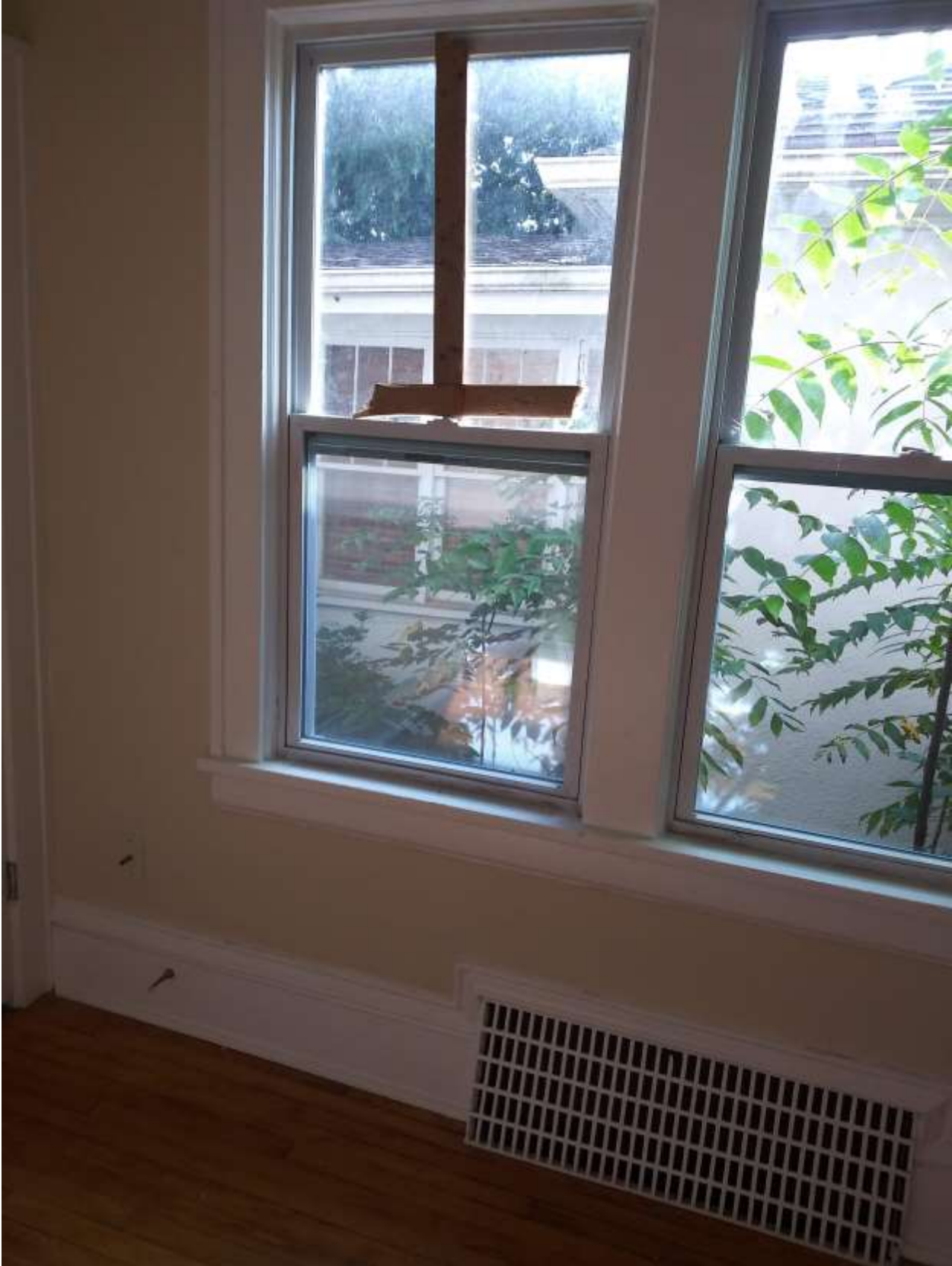
1842 Stillwater Ave. Photos sent by Lakisha Carpenter
