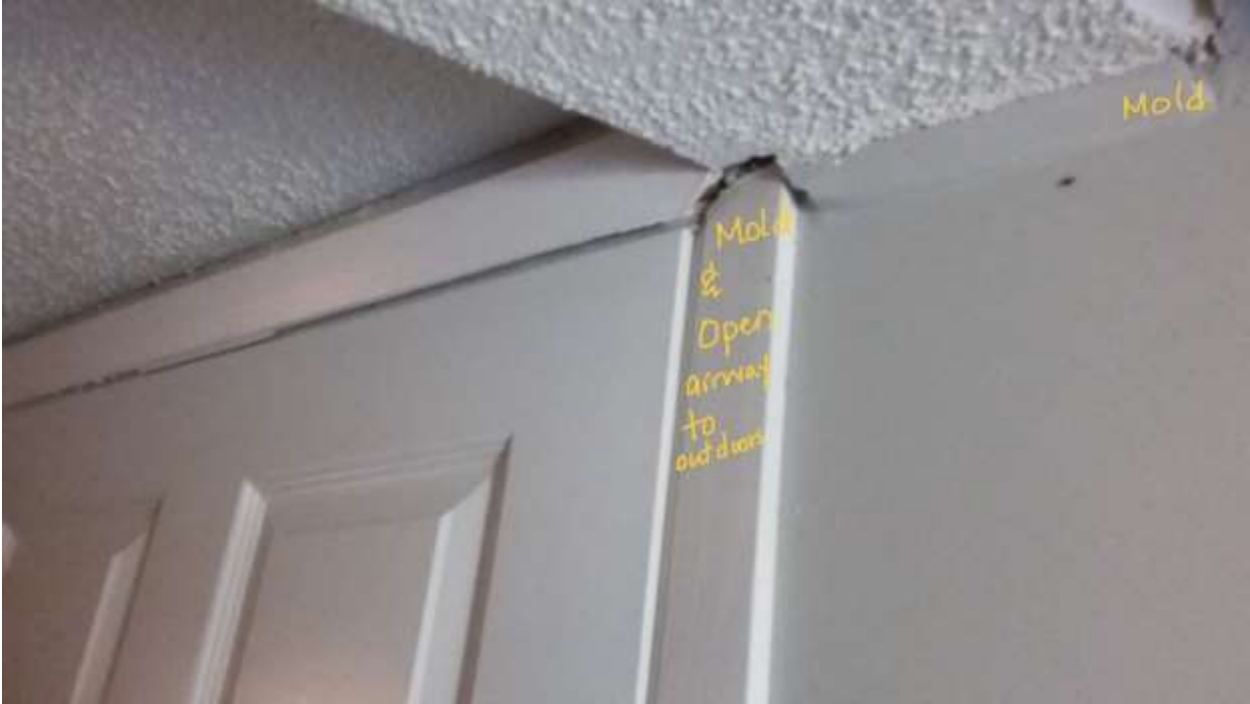
1842 Stillwater Ave. Photos sent by Lakisha Carpenter
