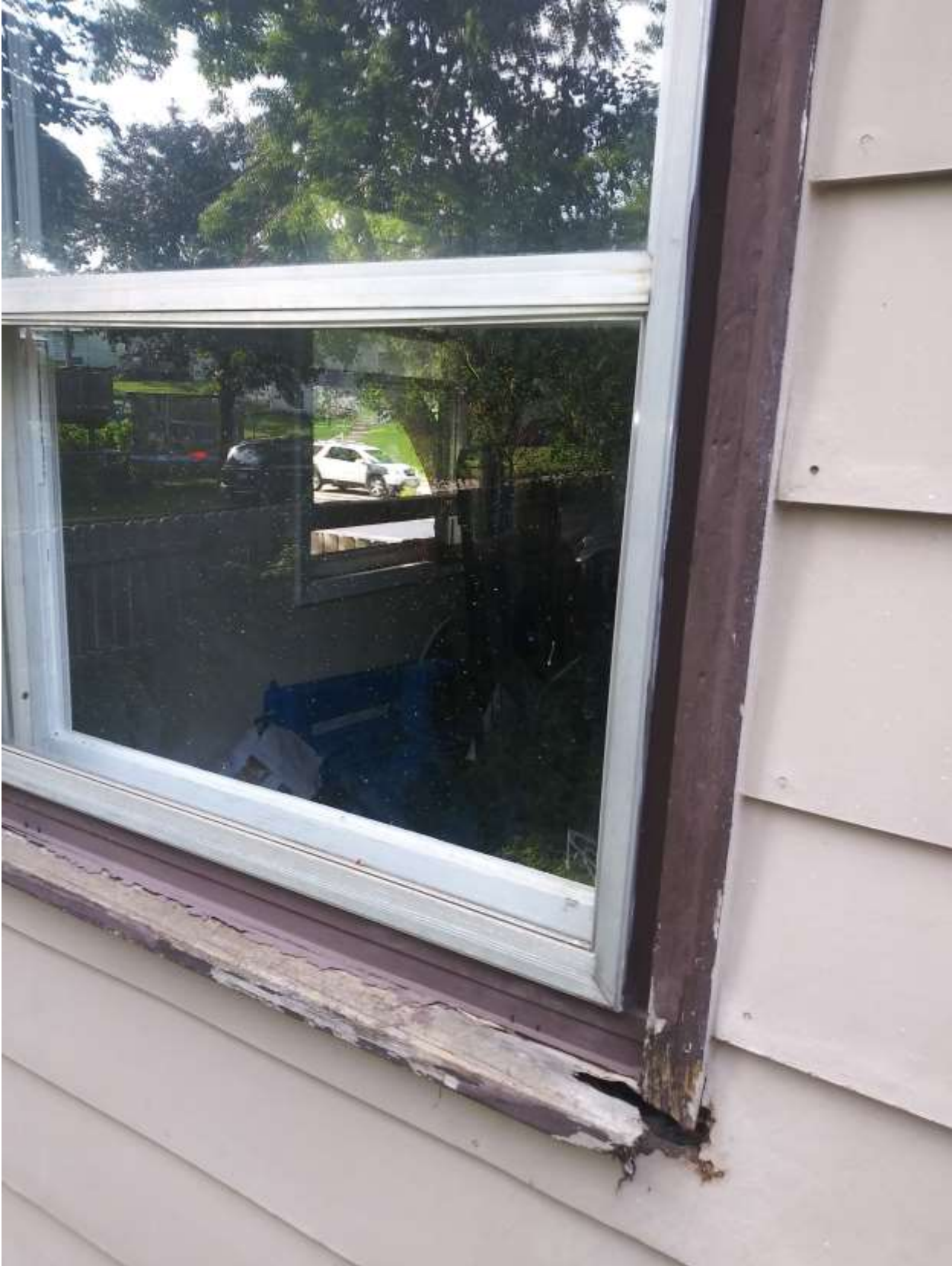
1842 Stillwater Ave. Photos sent by Lakisha Carpenter
