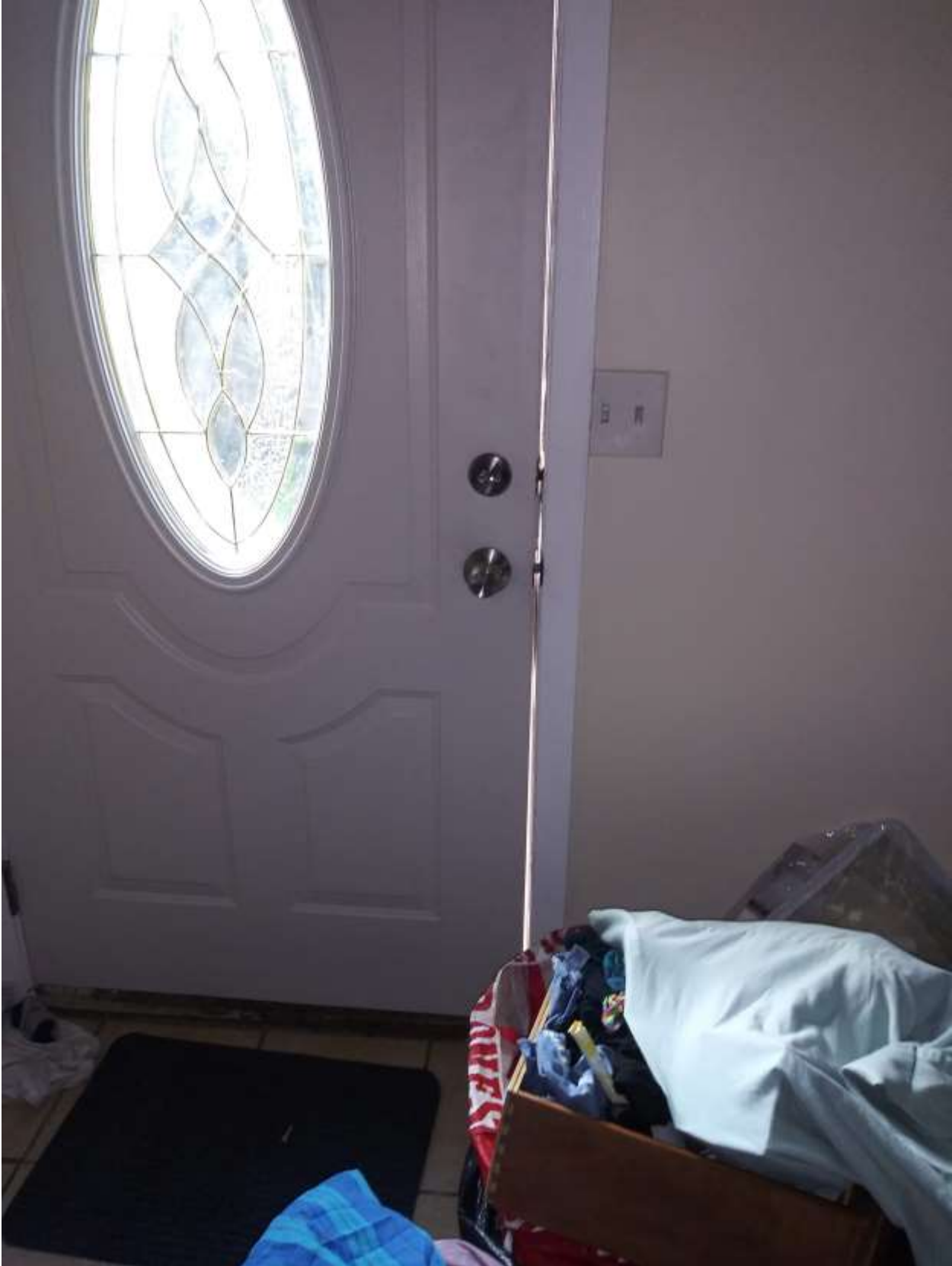
1842 Stillwater Ave. Photos sent by Lakisha Carpenter
