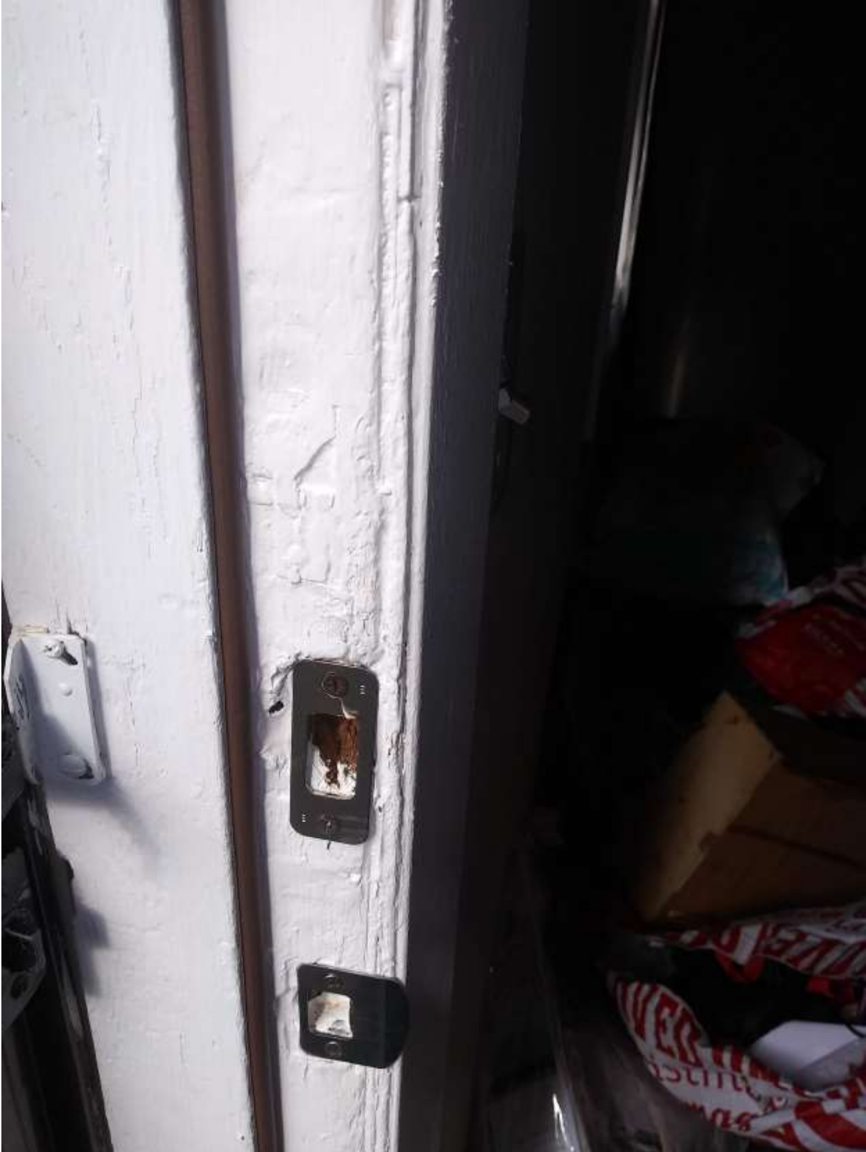
1842 Stillwater Ave. Photos sent by Lakisha Carpenter
