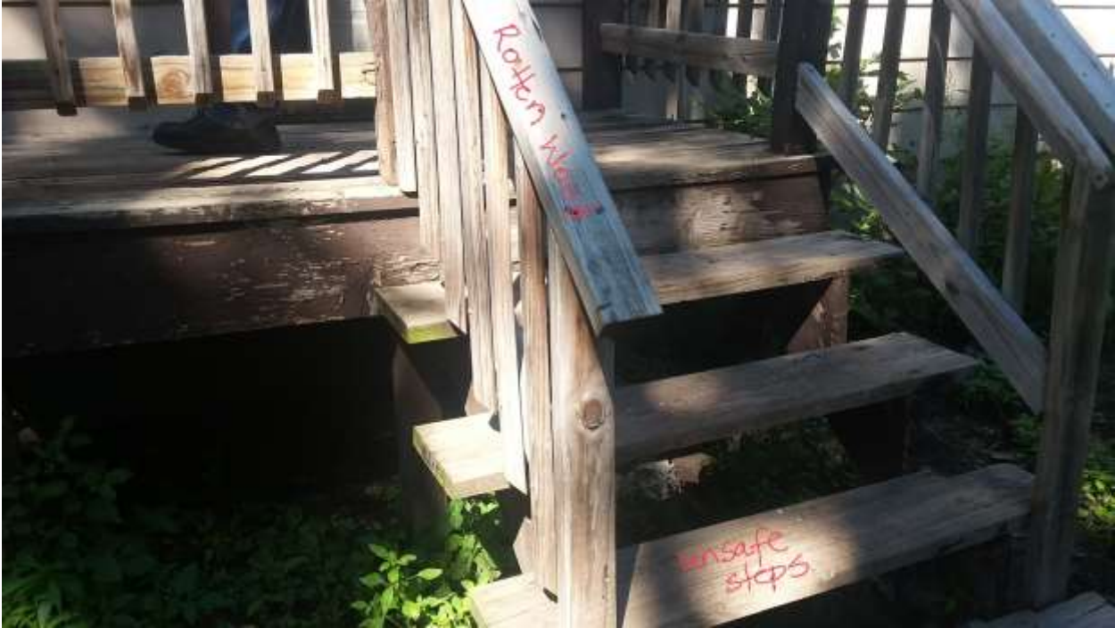
1842 Stillwater Ave. Photos sent by Lakisha Carpenter
