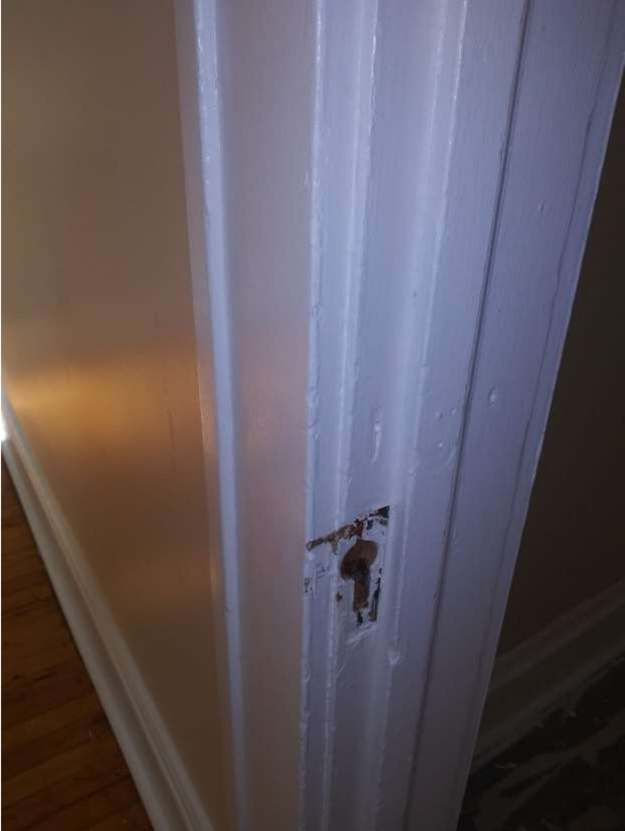
1842 Stillwater Ave. Photos sent by Lakisha Carpenter
