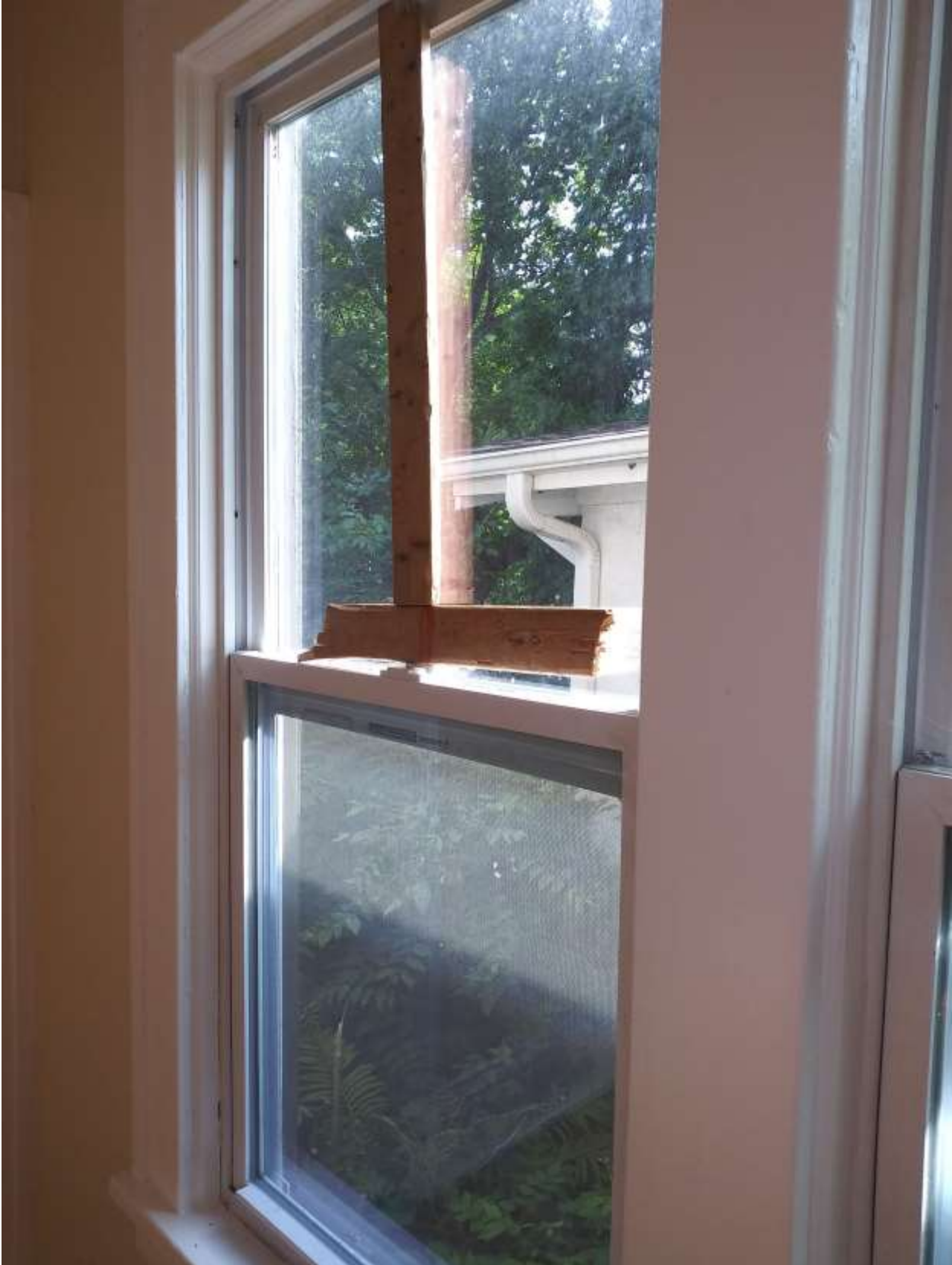
1842 Stillwater Ave. Photos sent by Lakisha Carpenter
