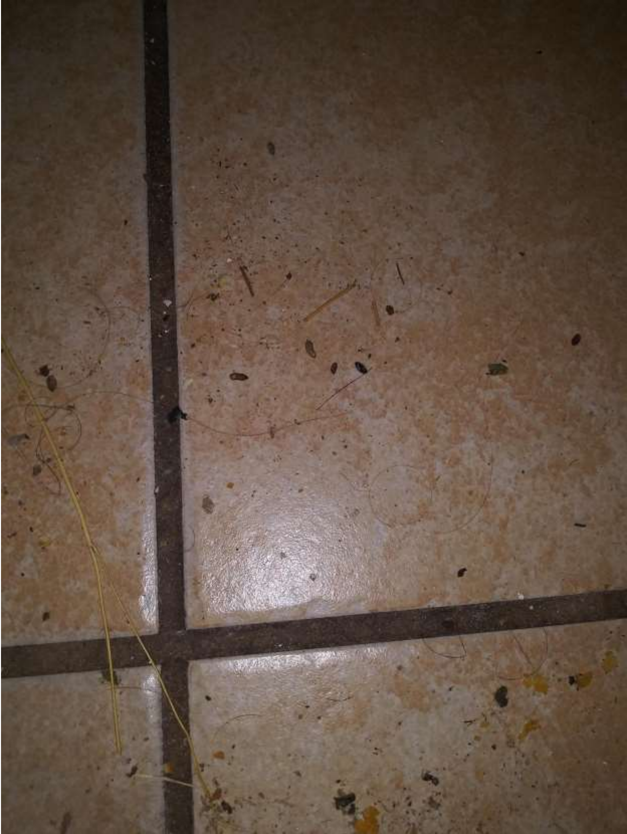
1842 Stillwater Ave. Photos sent by Lakisha Carpenter
