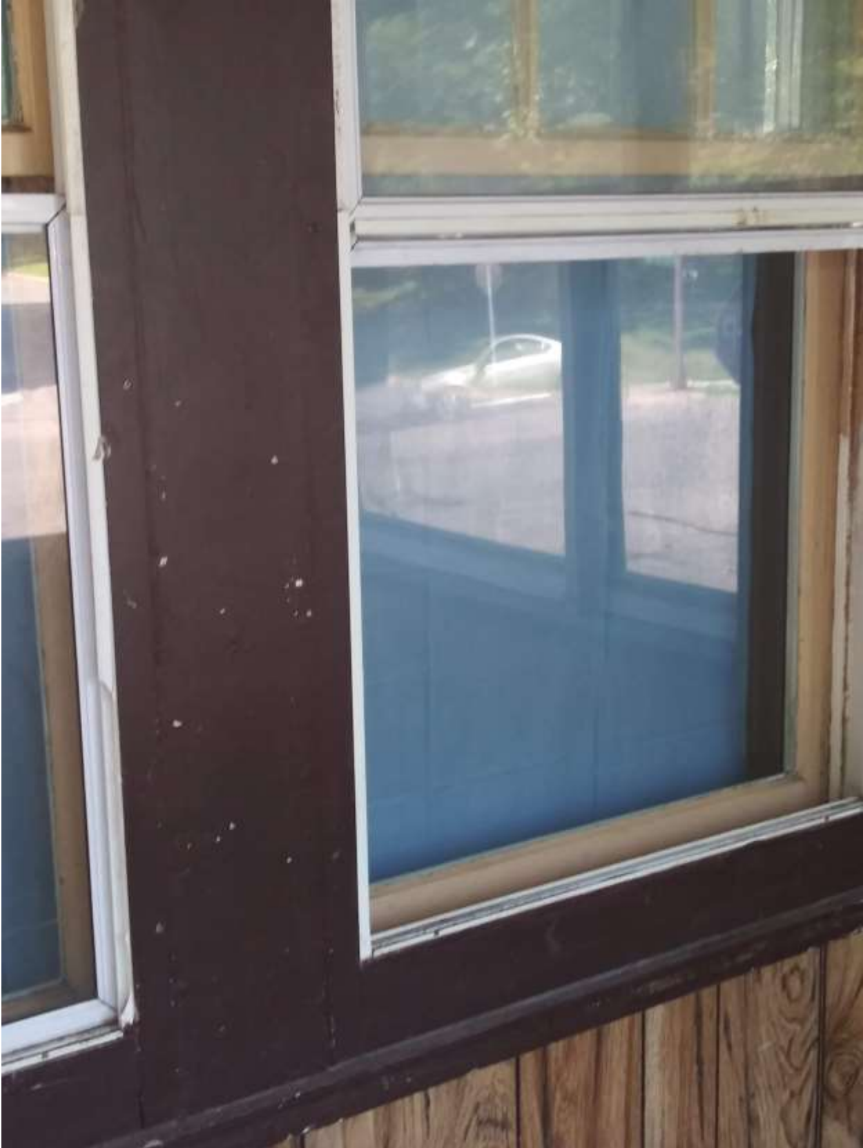
1842 Stillwater Ave. Photos sent by Lakisha Carpenter
