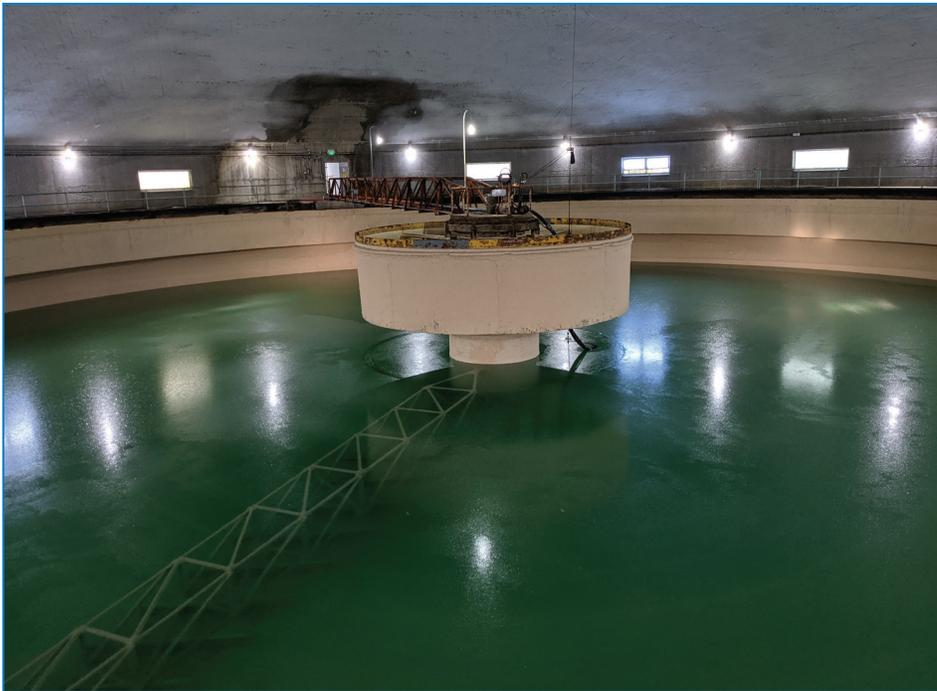
*Clarifier II starts to drain over the New Year's holiday weekend in preparation for the annual maintenance in clarifiers I and II and floc 3 this winter. The cold snap froze the water making it hard to drain.*
