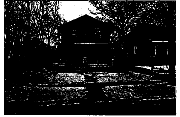
FRONT OF 1226 GOODRICH AVENUE CITY OF ST. PAUL, RAMSEY COUNTY, MINNESOTA
