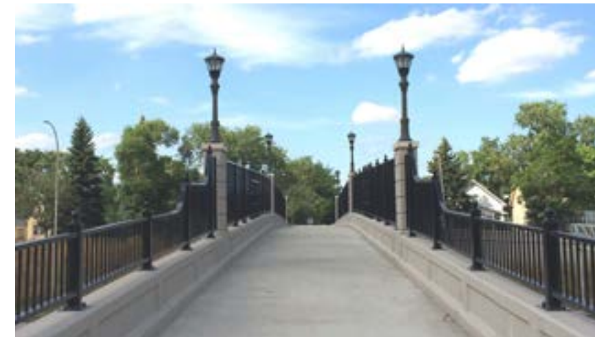
Figure 11: Pedestrian bridge over I-94 west of Downtown Saint Paul
