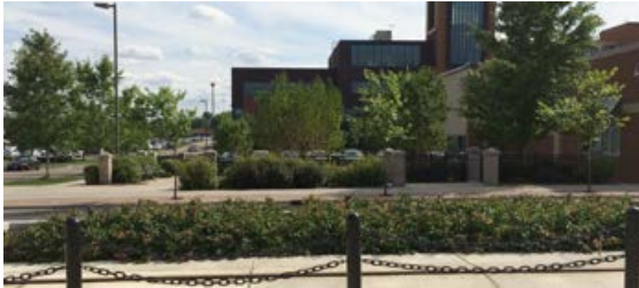
Figure 12: Stormwater treatment integrated with landscaping along the Green Line
