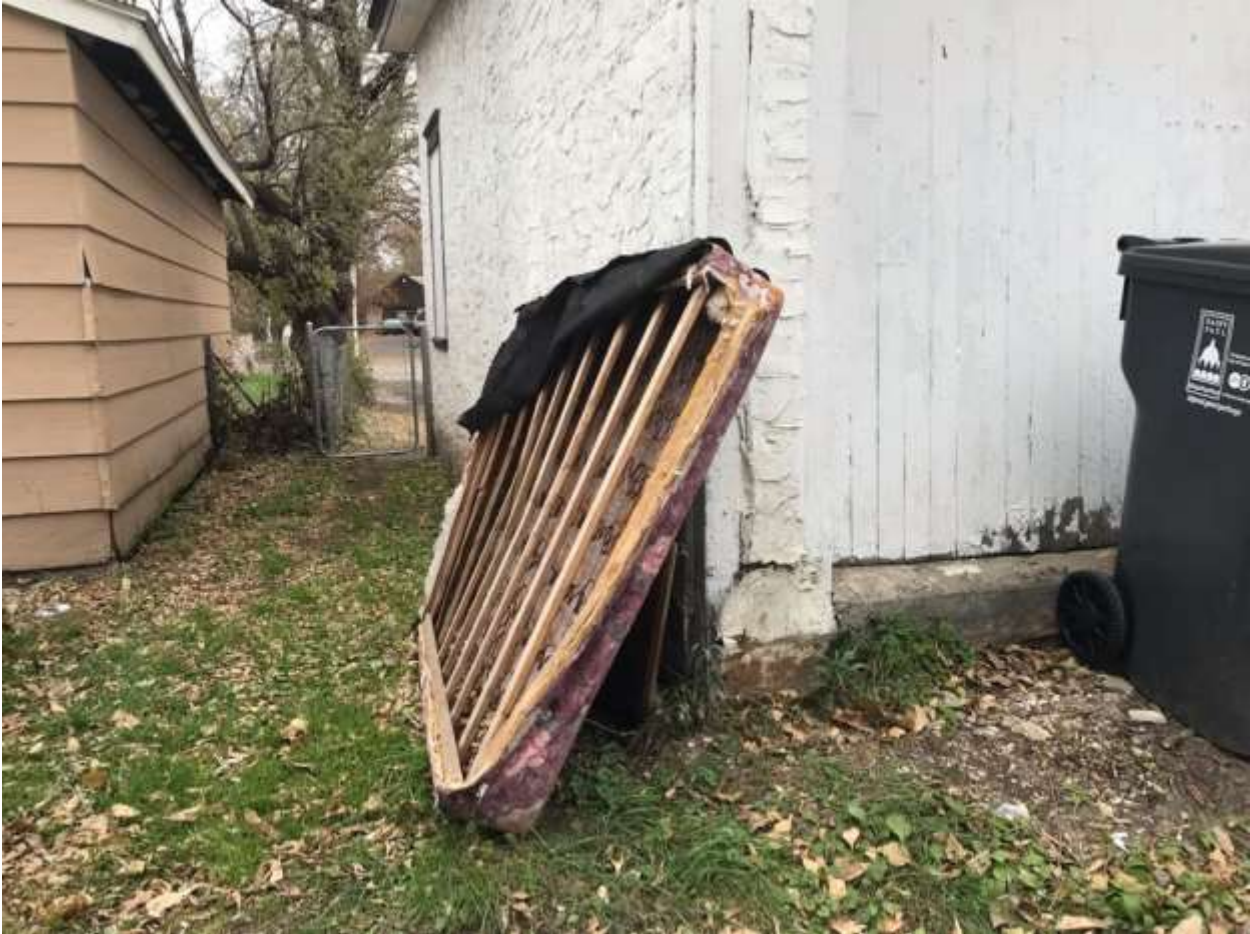
1252 Seventh St E.Photo upon reinspection.11-1-19
