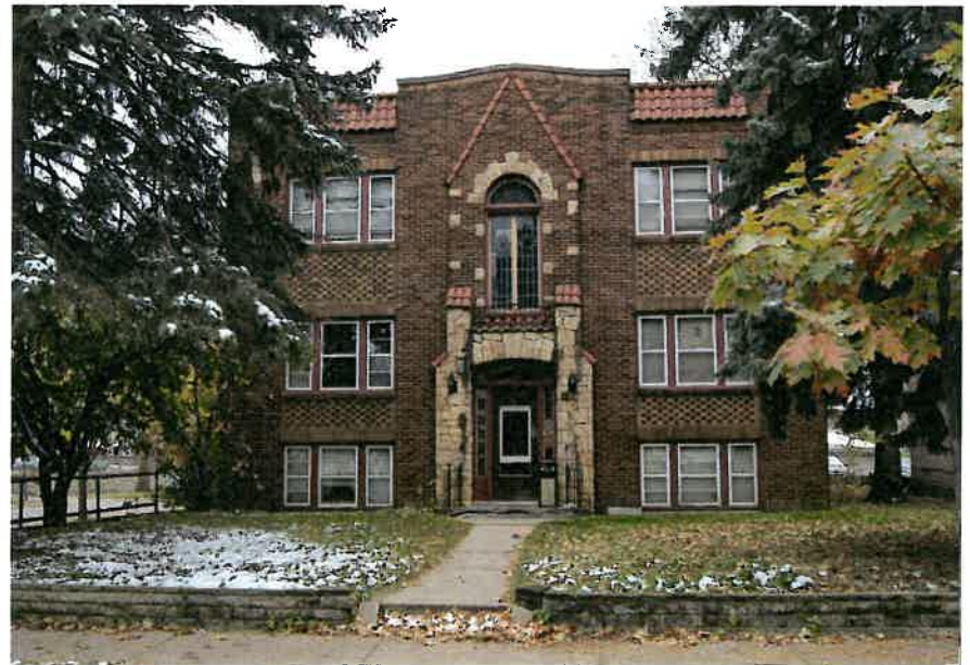
1630 Marshall (built 1929, at Fry Street)
