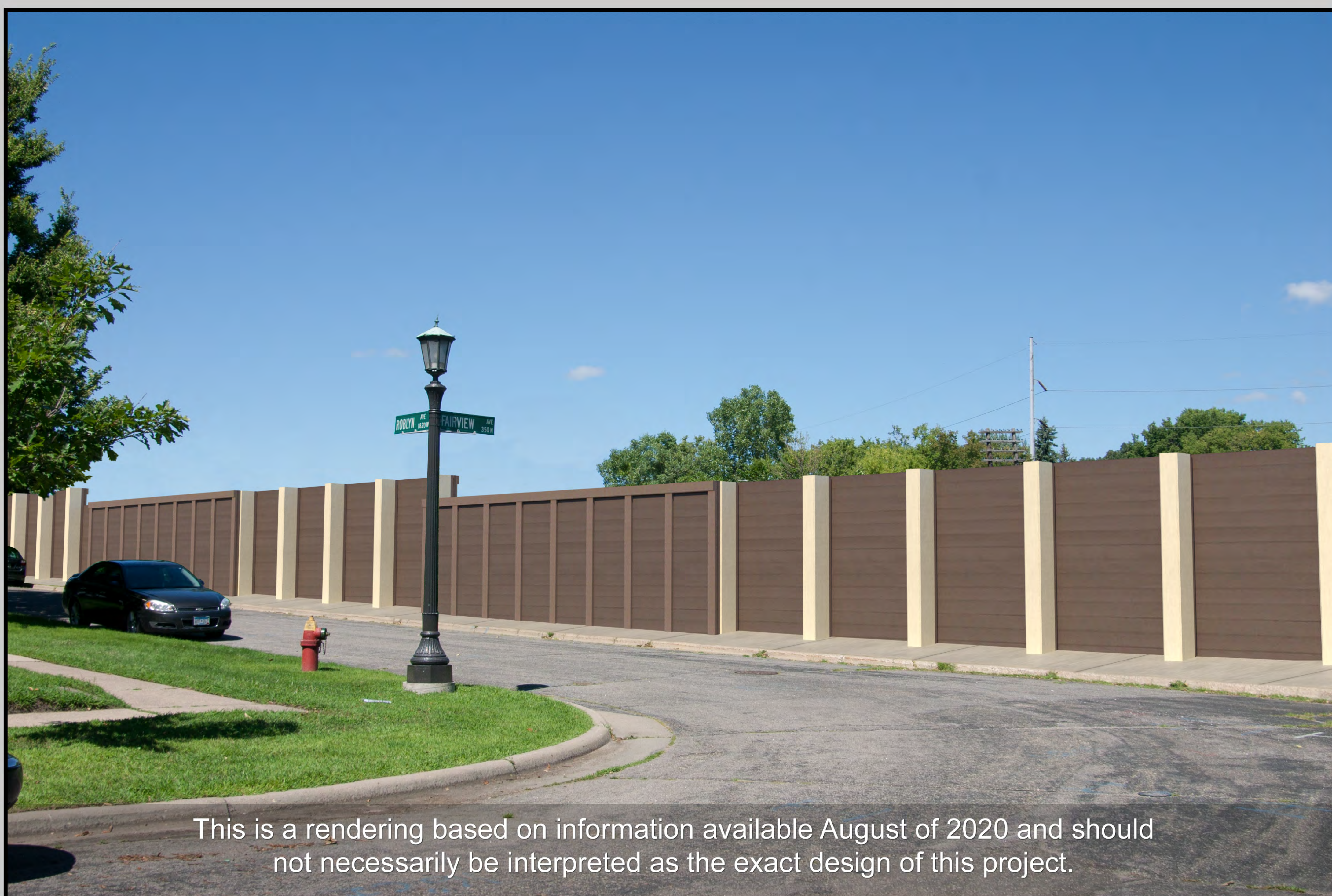
Proposed View - Construct 10' noise wall on existing retaining wall.
