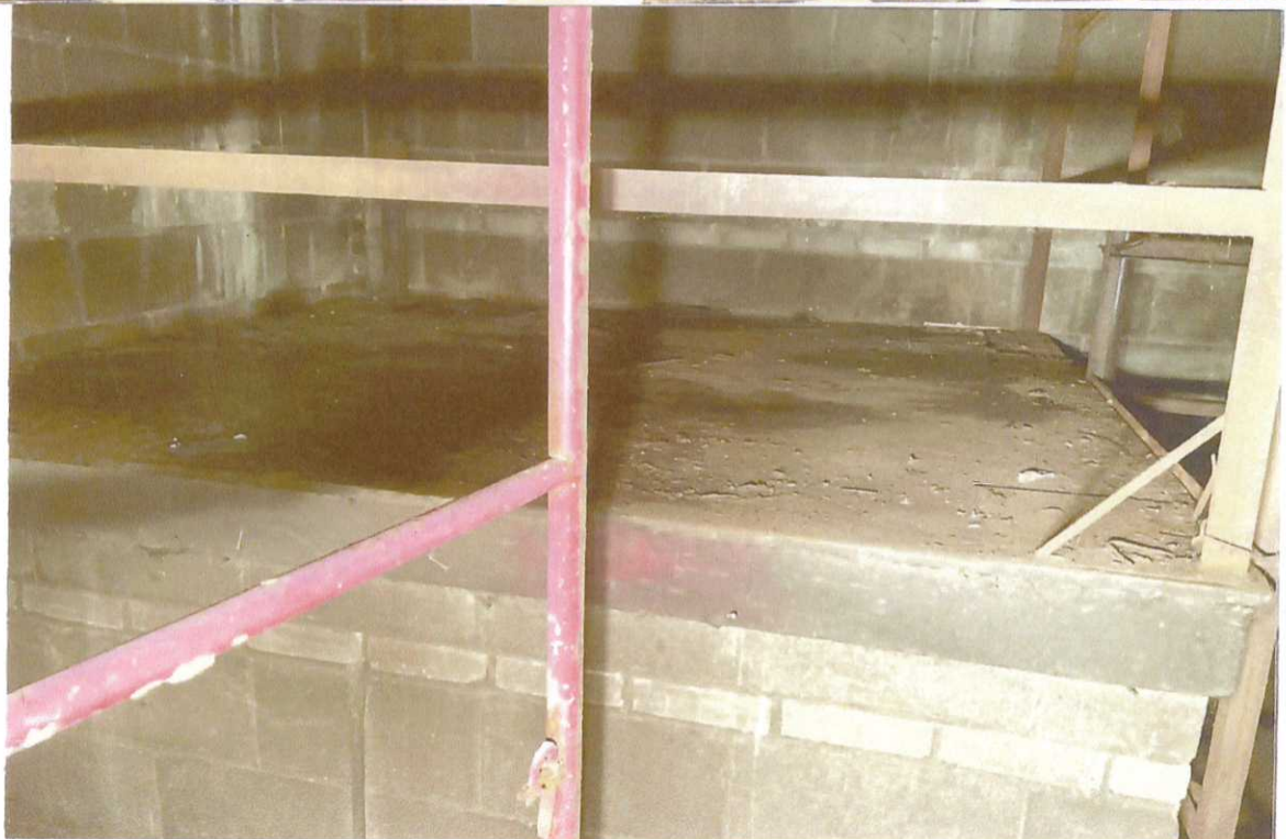
SW Mezzanine Cleared
