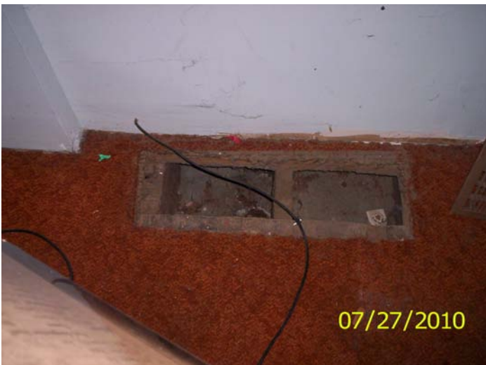
Open heating vent
